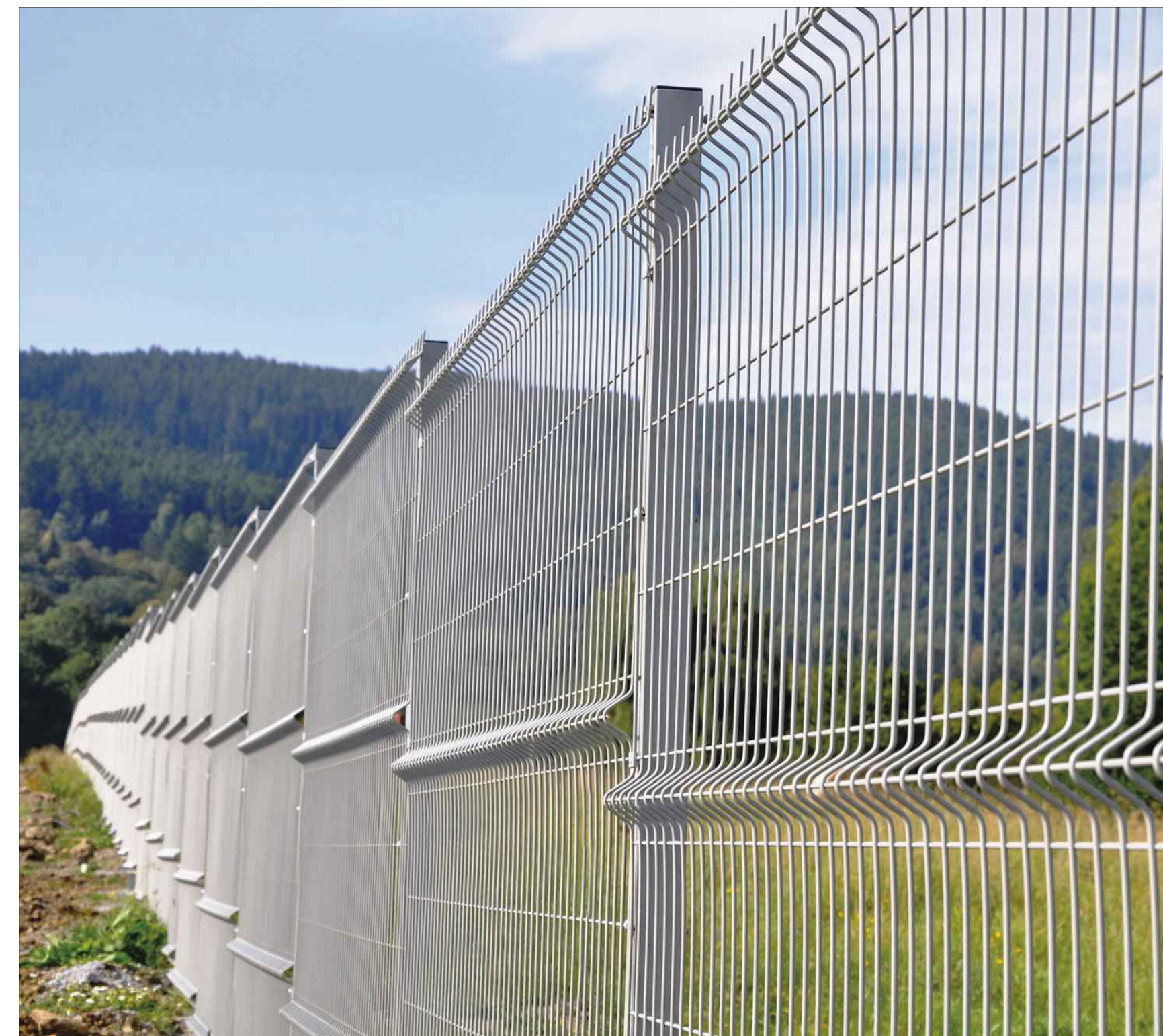
WELDED MESH FENCE EXAMPLE
