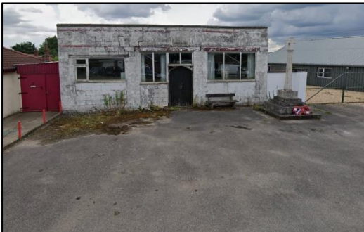
Site Photograph – front facade
