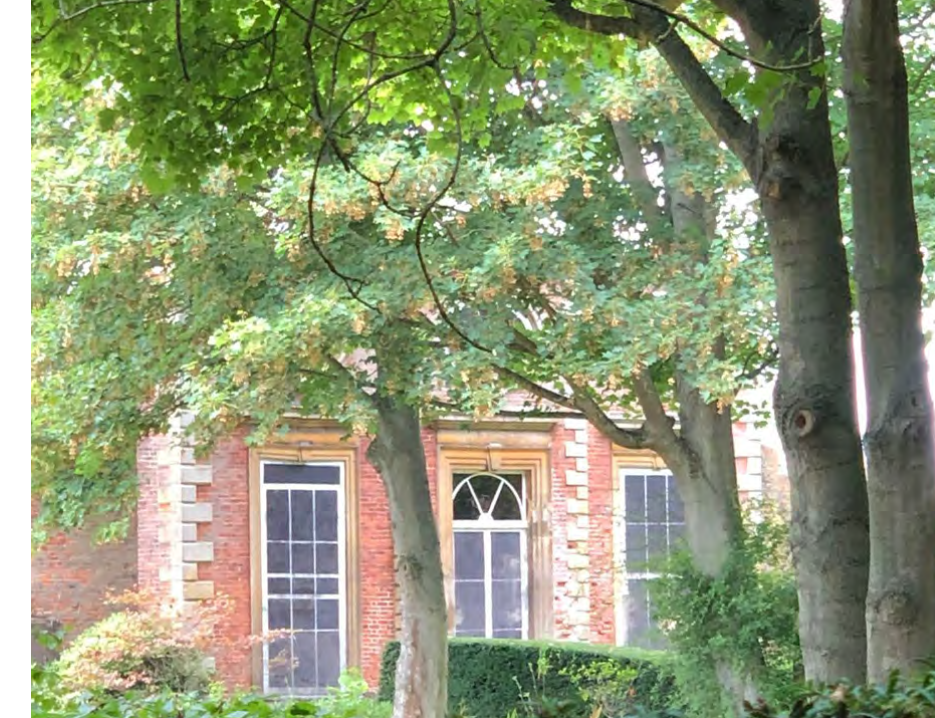
Glimpse view of the east elevation of The Pheasantry, through the mature trees taken from the footpath within the grounds of Nocton Hall.
