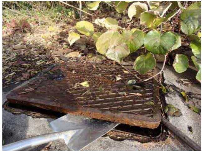
Water cistern removable cover. Lever tools were required to remove it.
