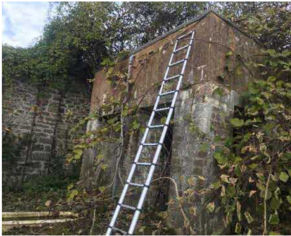
External masonry water storage cistern c. 3.5m tall.
