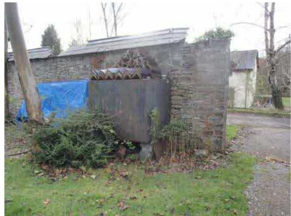
Disused steel oil tank at entrance. Clients wish to retain as a feature
