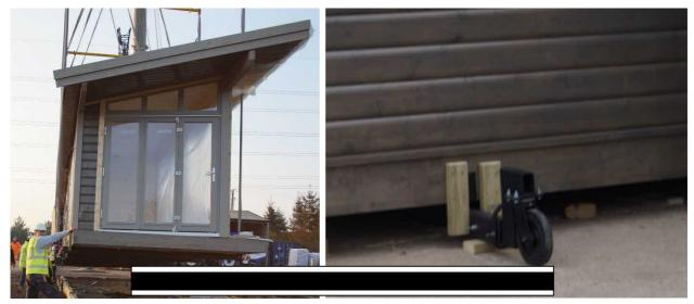
Due to the size of the proposed twin unit caravan, the road and site access complexities, independent assembly of the two individual sections will take place on site, they will then be moved into position with connecting as the final act.
