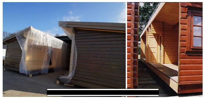
The process of assembly is identical whether undertaken offsite or onsite. The two sections of a twin unit caravan are independently assembled, they are then brought together by lifting or wheeling into position (see below), with the final act being connection of the two sections to form a whole.
