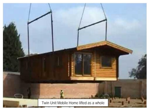
Due to the size of the proposed twin unit caravan, the road and site access complexities, the independently assembled sections will be wheeled into position with the connection being the final act.
