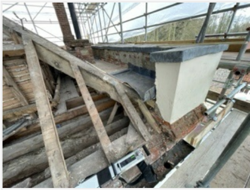
Figure 8: Showing northwesterly hip rafter.
