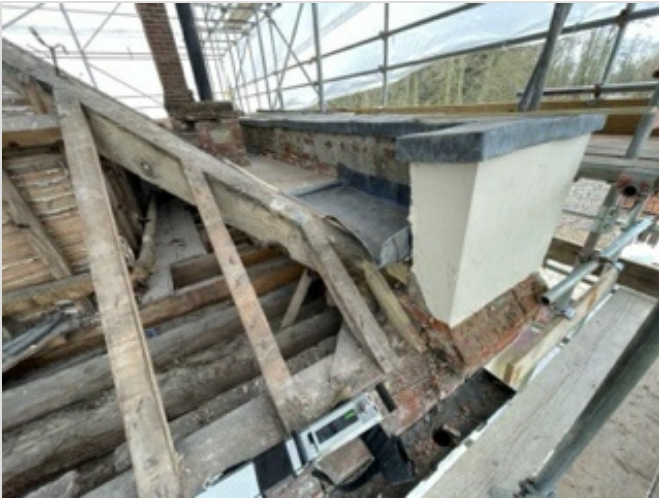
Figure 8: Showing northwesterly hip rafter.
