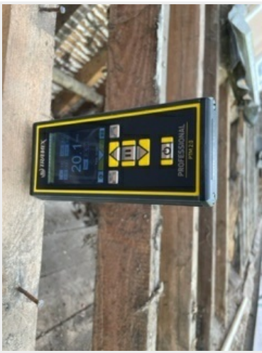
Figure 5: Recording wood moisture content.
