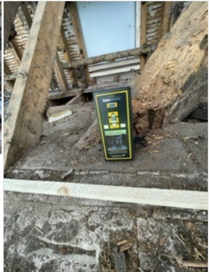
Figure 4: Recording wood moisture content.
