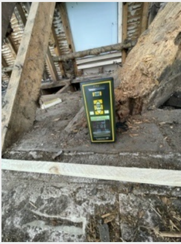
Figure 4: Recording wood moisture content.
