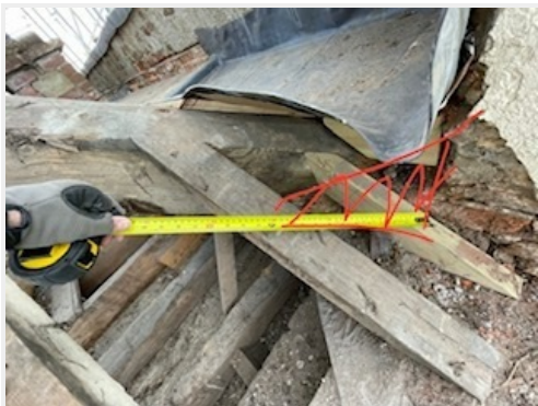
Figure 10: Showing position of decay identified thus far.
