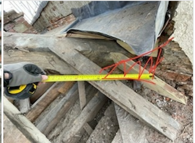
Figure 10: Showing position of decay identified thus far.
