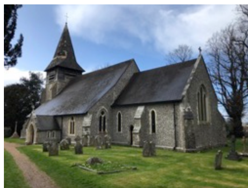
Present day appearance. The aisles, belfry and spire were reconstructed, and buttresses added, in the C19.
