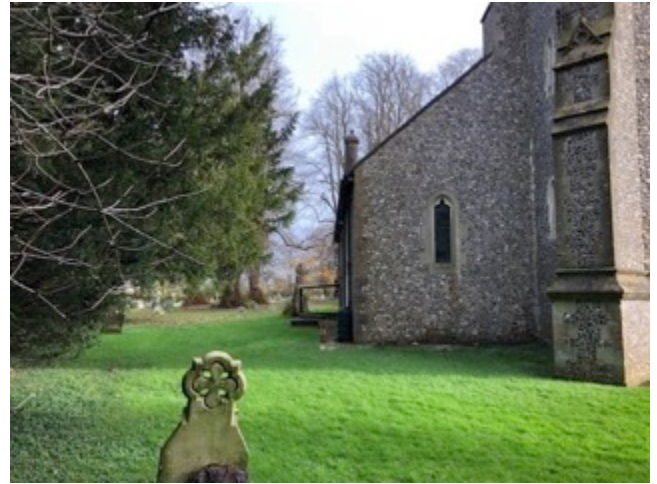
2 West end of the North Aisle. The extension would project into the space on the left of the building. There would be enough clearance for the public footpath to pass alongside.
