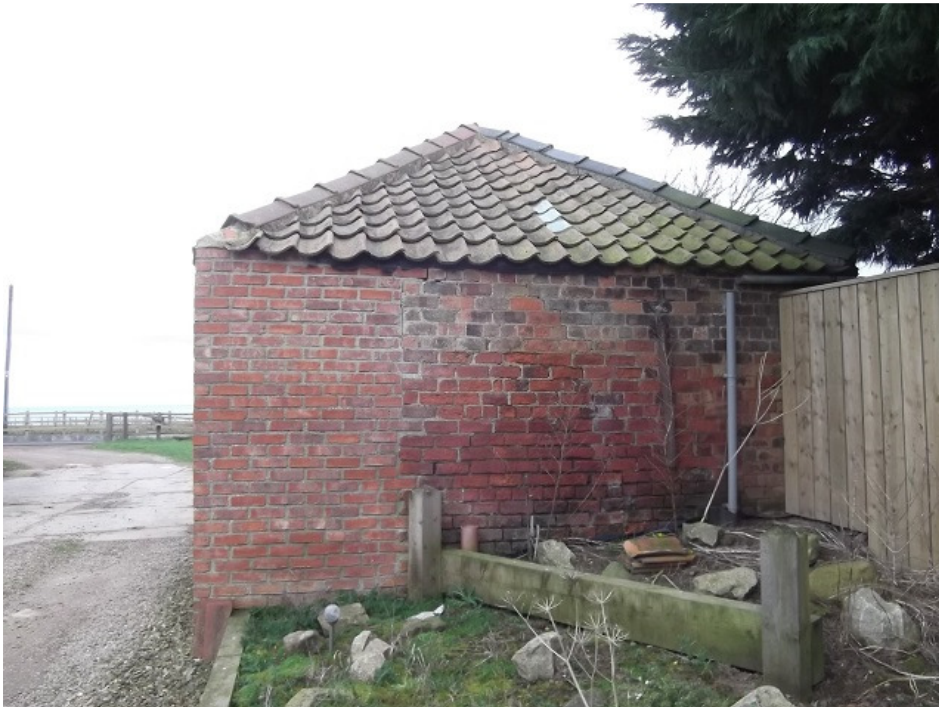
Plate 3. Looking at the west gable of the study building.
