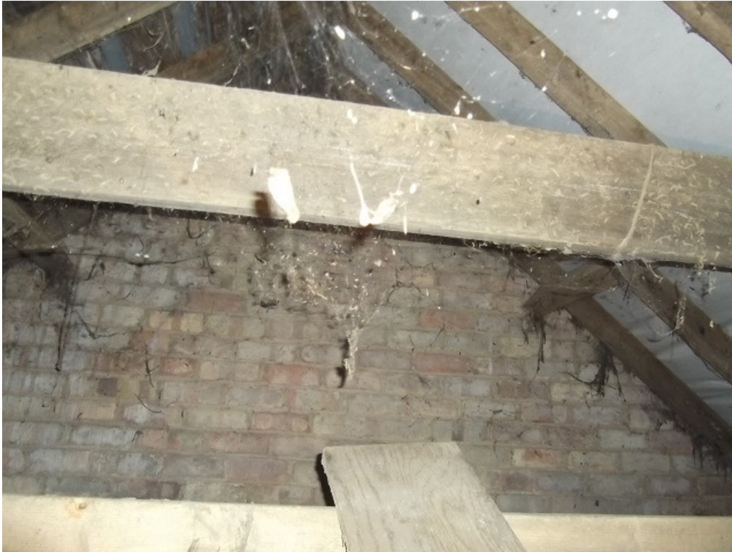
Plate 6. The accessible section of the roof void.
