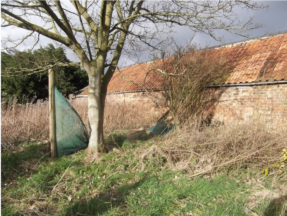
Plate 2. Looking at the south elevation of the study building.
