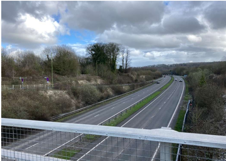
Viewpoint 7 - Taken from the bridge over A41. Site cannot be seen.
