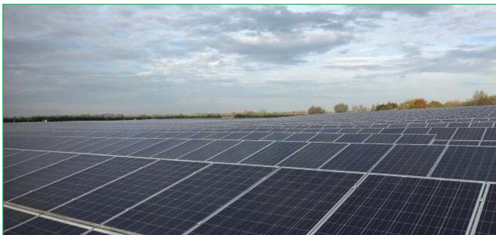
Figure 6 - Typical View of Arrays with Joints which Distribute Runoff
