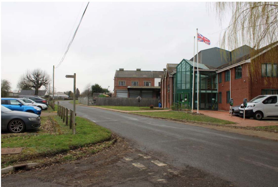
Plate 25: View north showing the extent of the For Farmers complex along Mill Road, with further modern development to the west of the site beyond
