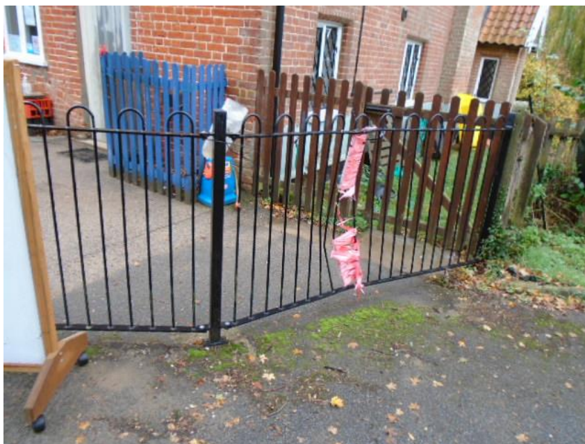
Example of fencing to be removed
