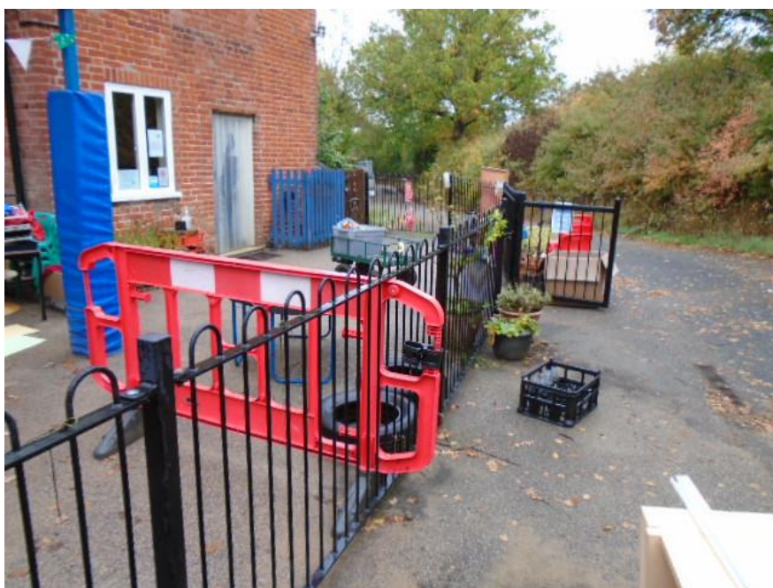
Example of fencing to be removed
