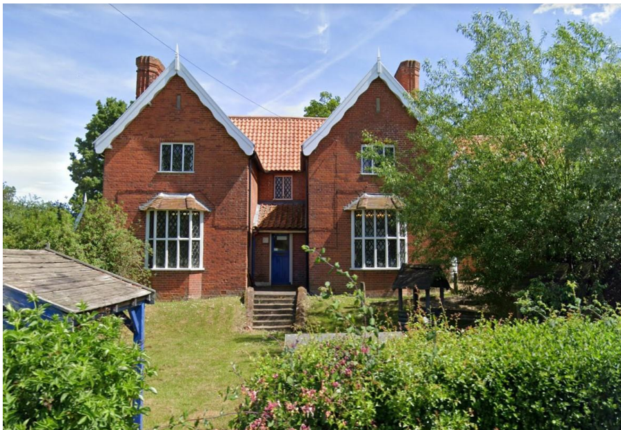
West elevation of School House
