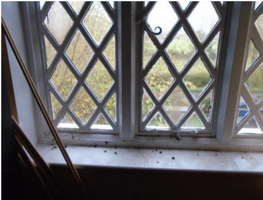
Upper floor Room 21 showing window facing west to receive secondary glazing
