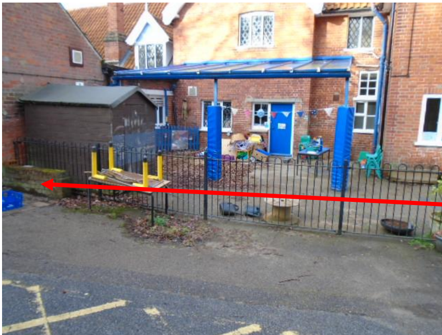
East elevation of School House showing canopy to be removed
