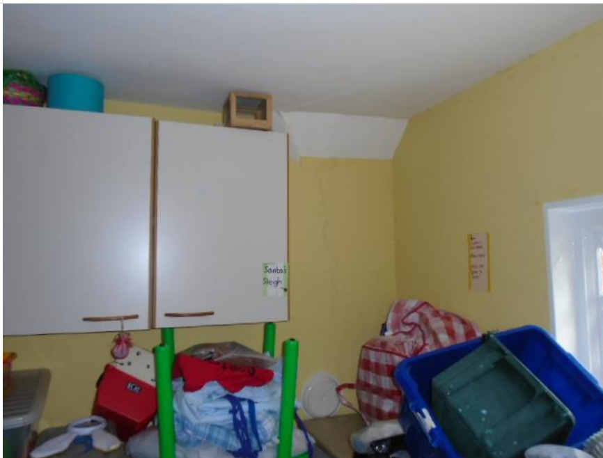
Upper floor Room 22 to be refurbished
