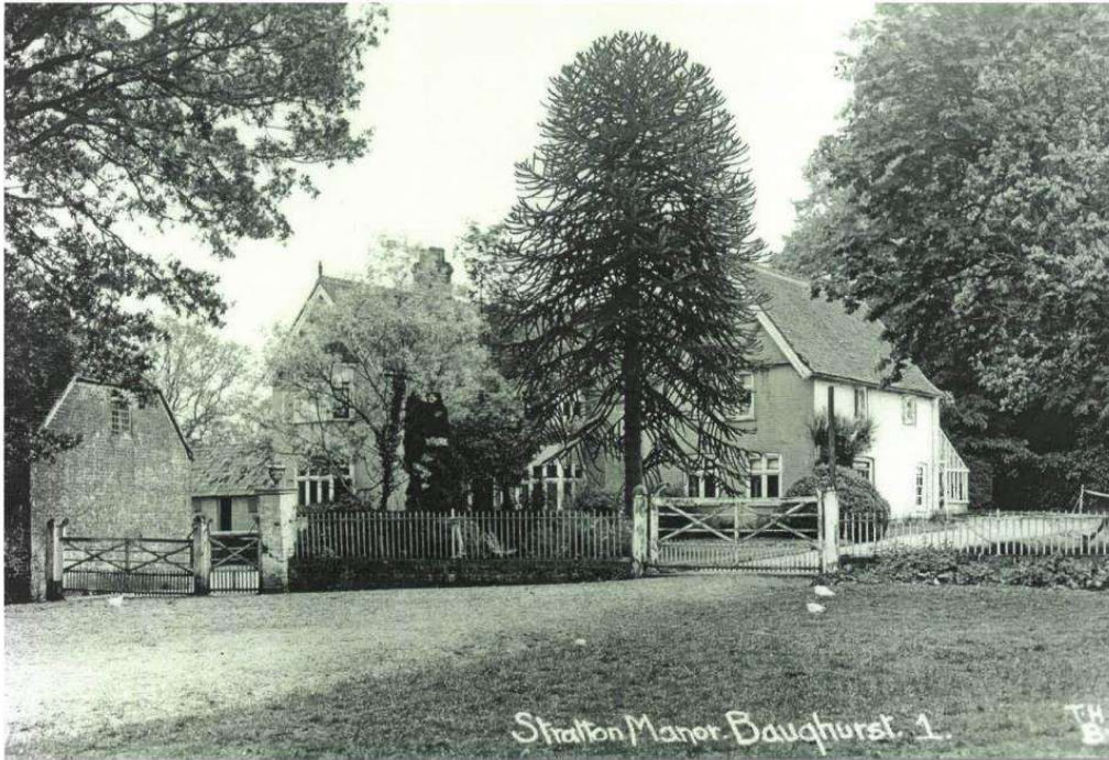
Photo of Stratton Manor, possibly taken about 90 years ago. This shows the half-hipped end of the building on the application site as it appeared at that time. The ridge height of this original part of the building is estimated to be approx. 7.0m.
