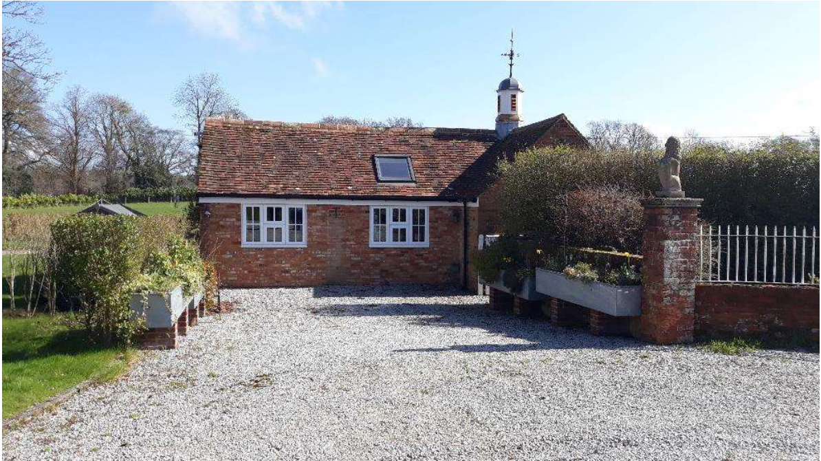
View of the existing Cottage at Stratton Manor, looking East
