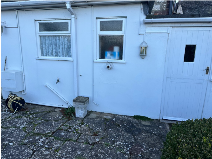
Existing extension to be demolished and replaced.
