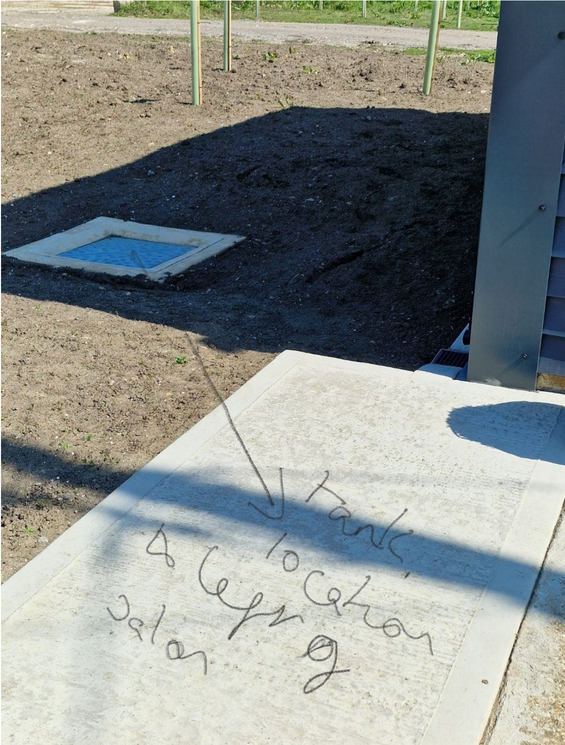
Grey water holding tank location. There is no foul waste from the building and the tank is emptied by a specialist firm when full.
