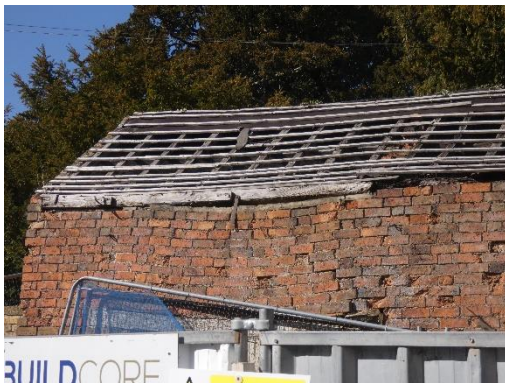
Figs. 5 & 6 Untiled roof at front
