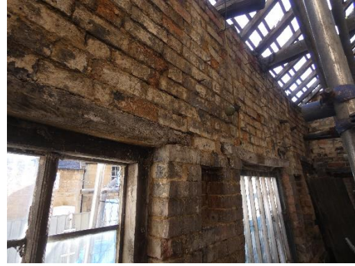
Figs. 13 & 14 Crack in internal wall (L) and windows (R)
