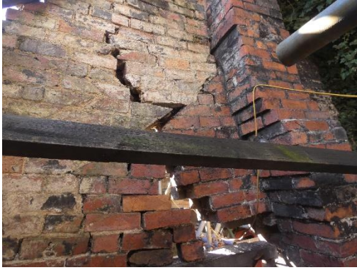
Figs. 13 & 14 Crack in internal wall (L) and windows (R)
