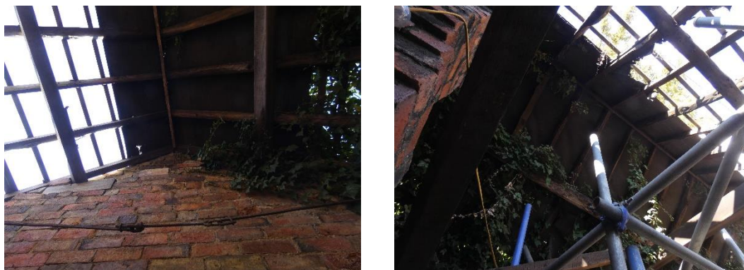
Figs. 11 & 12 Underside of roof of building
