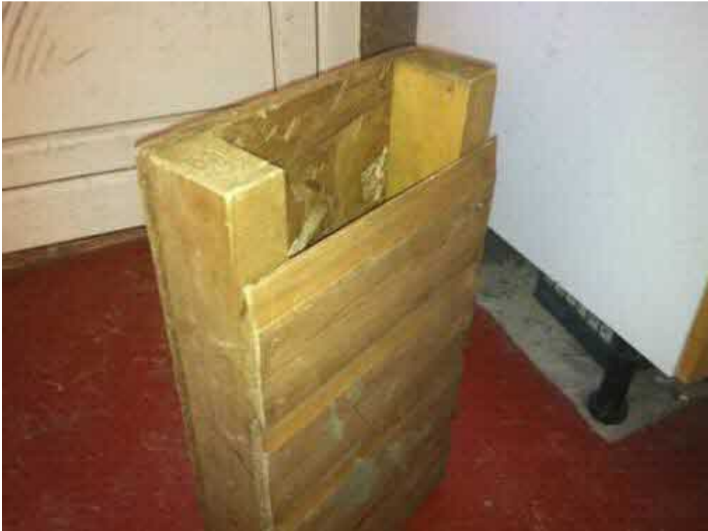
Section of the proposed stable construction. Timber stud construction with horizontal weatherboarding to the external face and finished internally with timber sheeting, such as plywood or OSB
