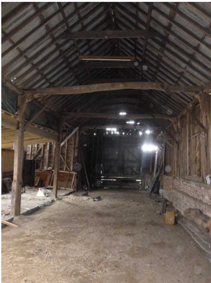
Original Interior of barn
