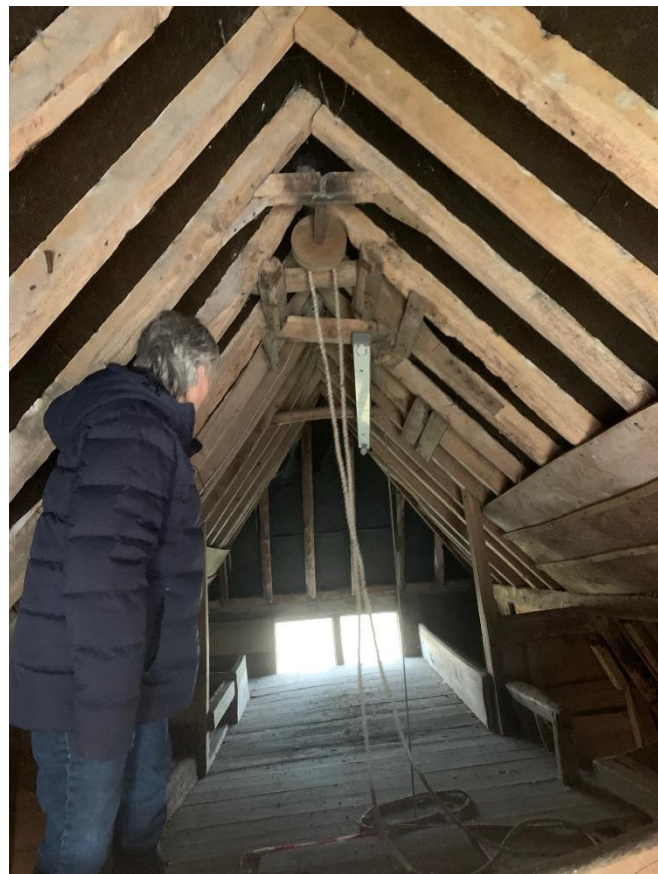
The Hoist pulleys and mechanism seen here with the owner of the Mill will be retained as part of the refurbishment plans. However, the upper floor of the bin floor will be removed together with some of the grain bins to facilitate the new layout. Hoppers will be retained where possible and an illustrative graphic with technical description of the bin floor mounted nearby on the wall.
