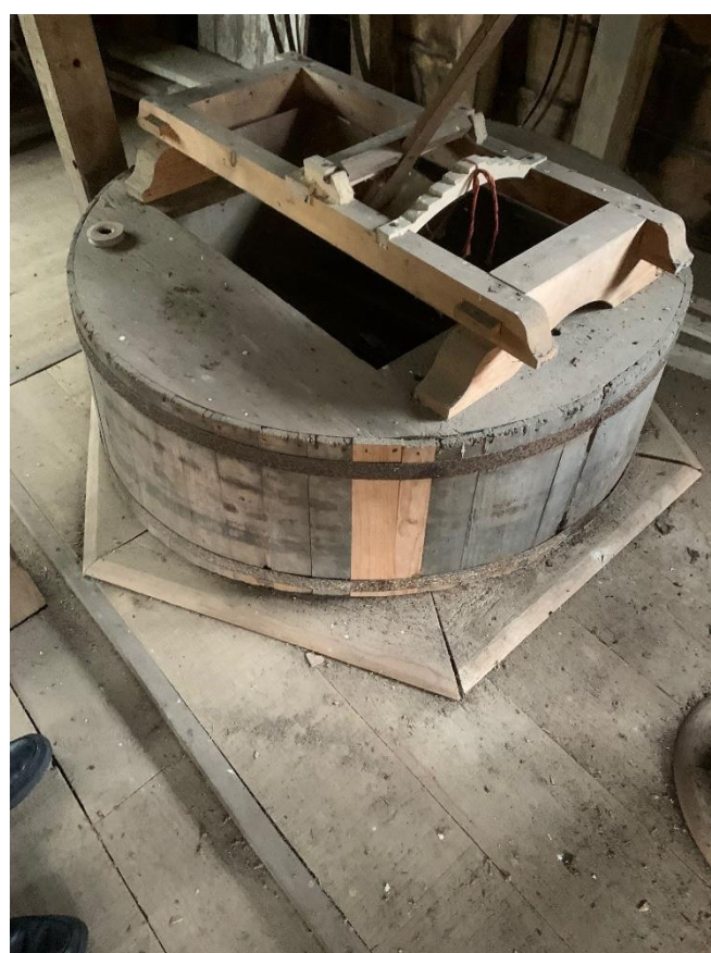
The Damsel, Horse, and Shoe containing the Millstones. This is where the grain would have been fed from a hopper into the shoe, which is vibrated by the damsel, shaking grain into the centre of the runner stone. - All to be retained and refurbished.
