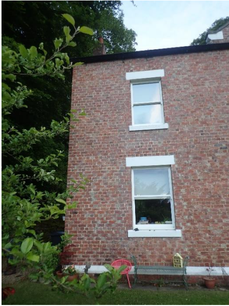
House, northwest aspect, showing bonded brick walls
