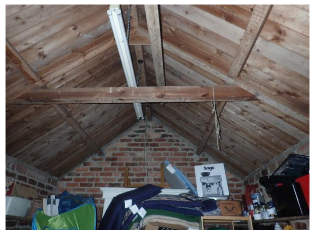
Crevices below the slate on the garage
