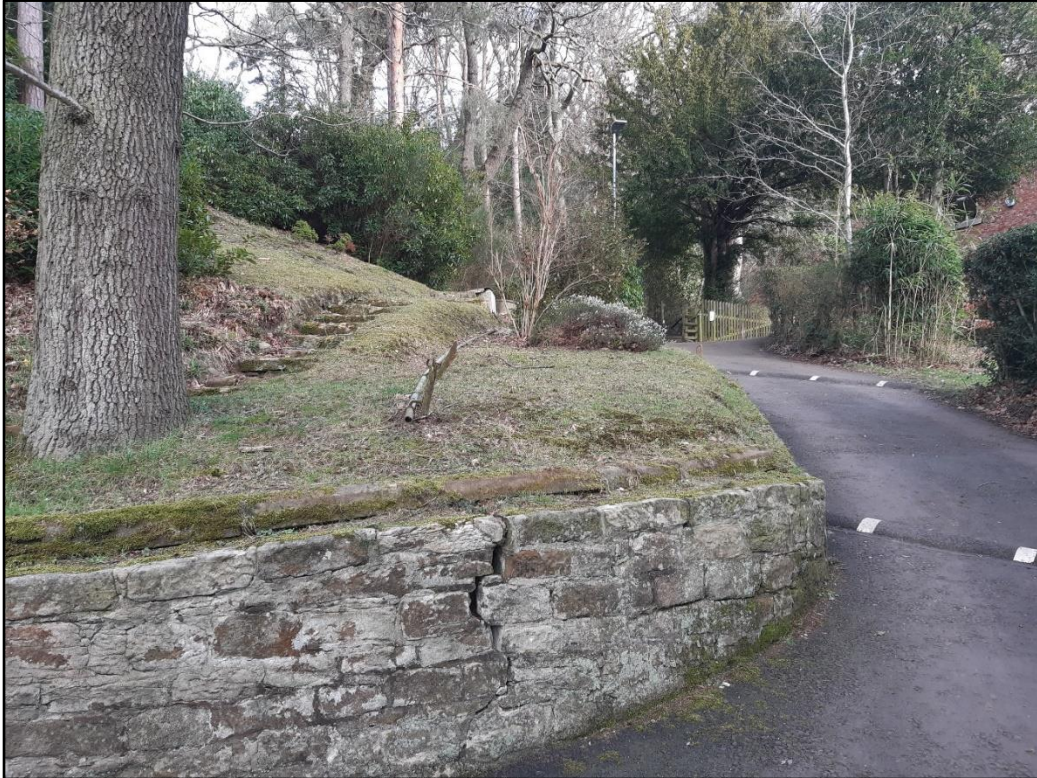
Figure 4 – The proposed location of the detached garage, to the rear of the oak in the foreground
