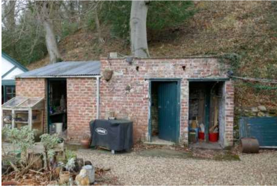
Figure 2: Existing outbuildings to be incorporated into the proposals
