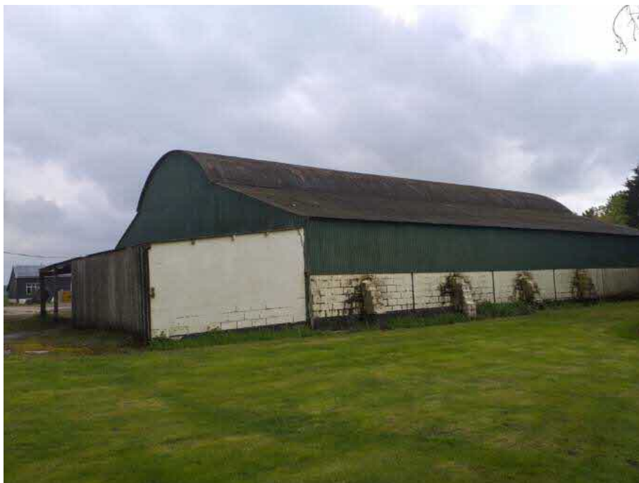
Building 3 viewed from north west
