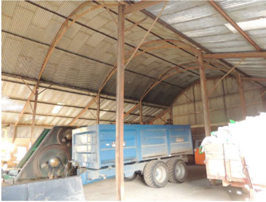
Building 3 interior had no features that might be occupied by bats
