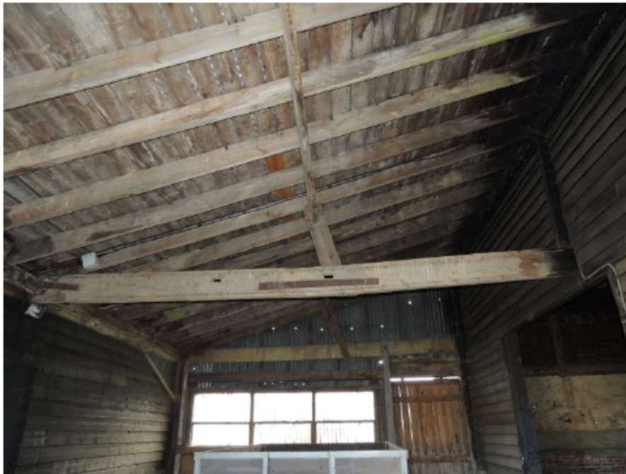
Interior of building 8 storage area
