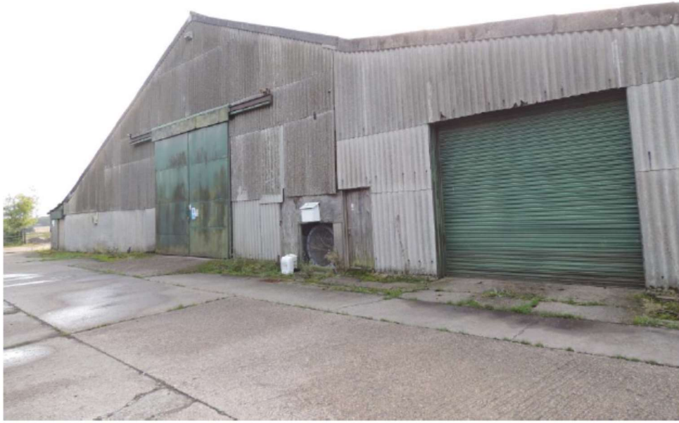
Photo 5 north western elevation
