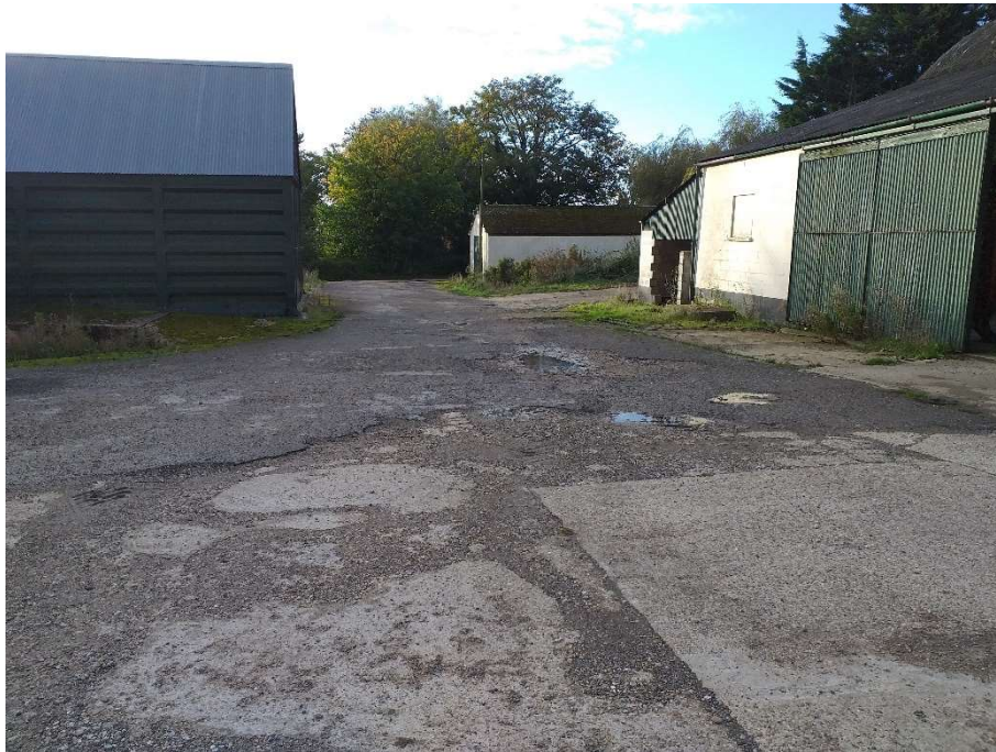
Hard standing yard section of site looking south
