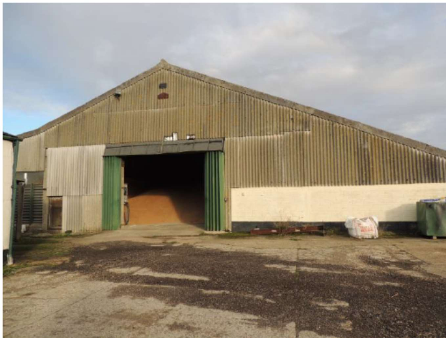
Buildings 1 & 2 south eastern elevation
