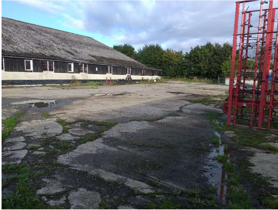
View across yard looking north west
