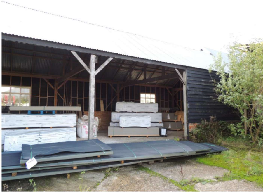
North west elevation of building 7
