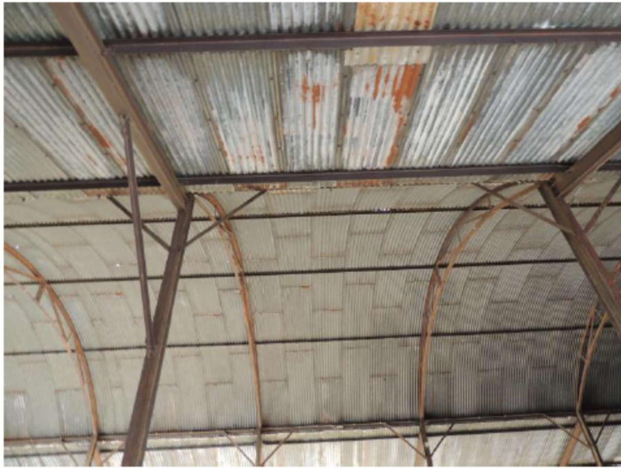
The roof had no features that might be occupied by bats
