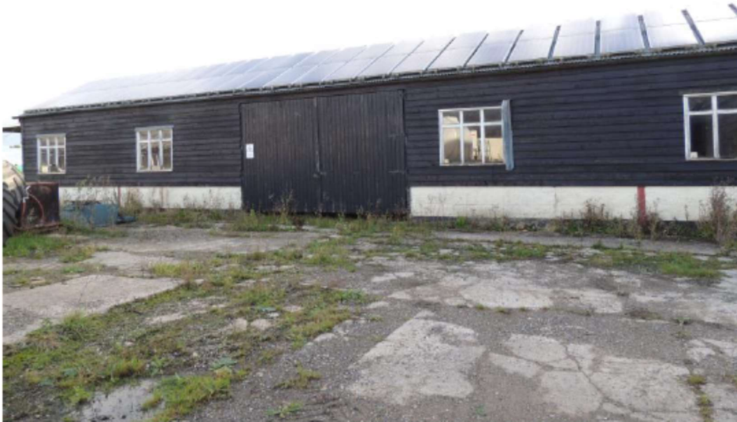
Building 5 south western elevation
