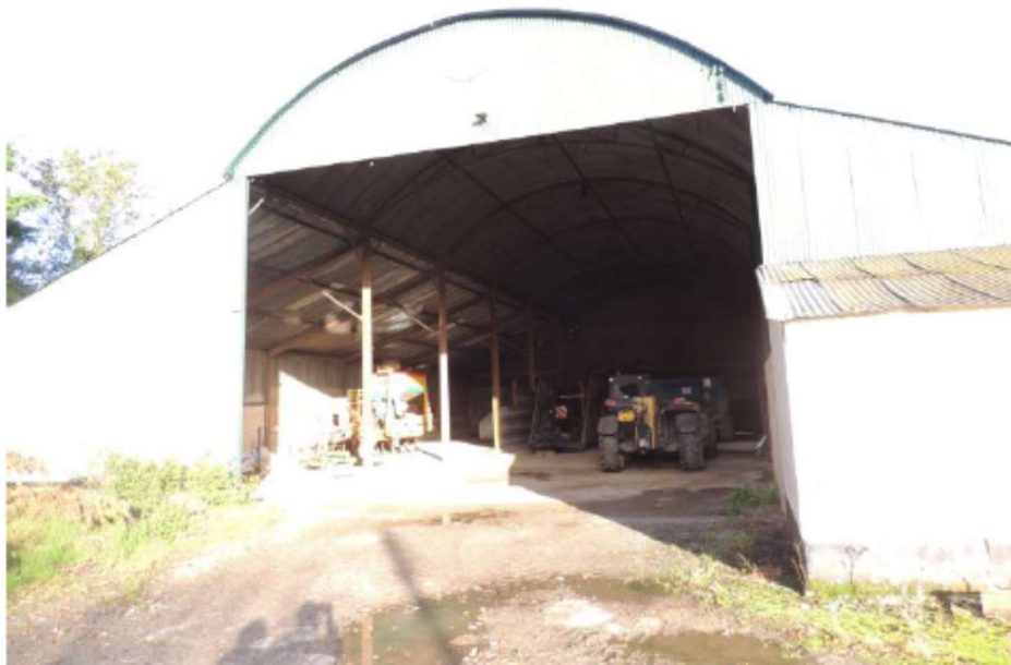
Building 3 south eastern elevation
