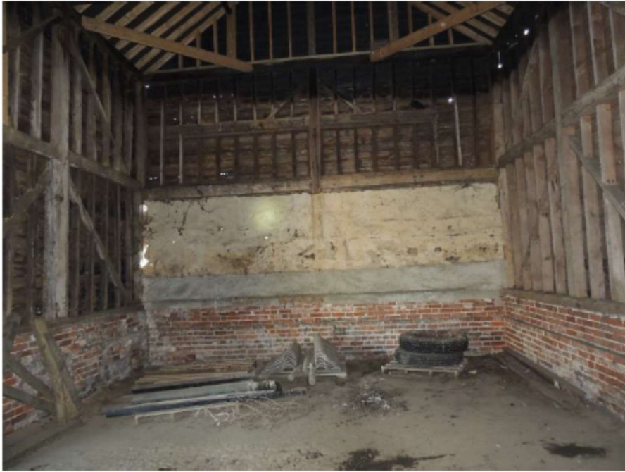
Interior of barn section of building 8
