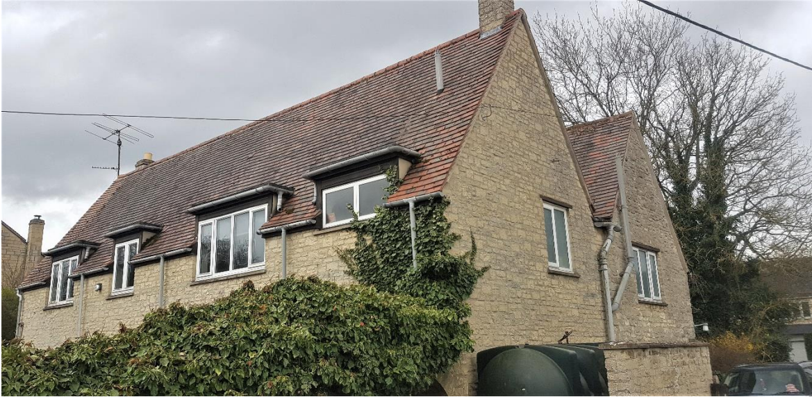
03 – Rear and side view of the existing dwelling, 101 Abingdon Road
