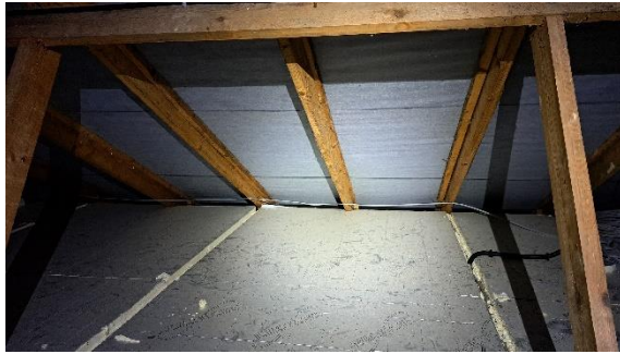
Photo 10 Interior View of loft space in area of extension
