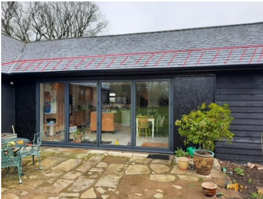
Photo 1 Section of Roof to be removed in the construction of the proposed extension (roof tiles to be removed indicated by red hatching)
