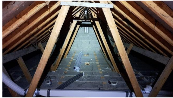
Photo 11 Interior View of loft space in area of extension.
