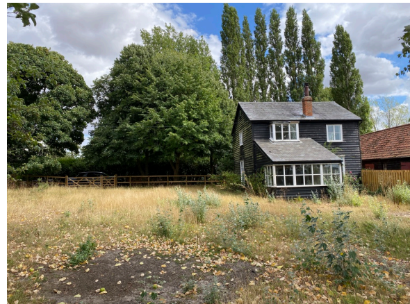
West elevation and garden
