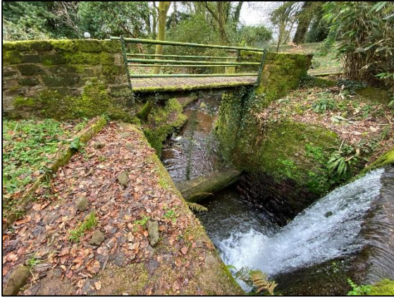
Plate 3: View from weir (facing south-east)
