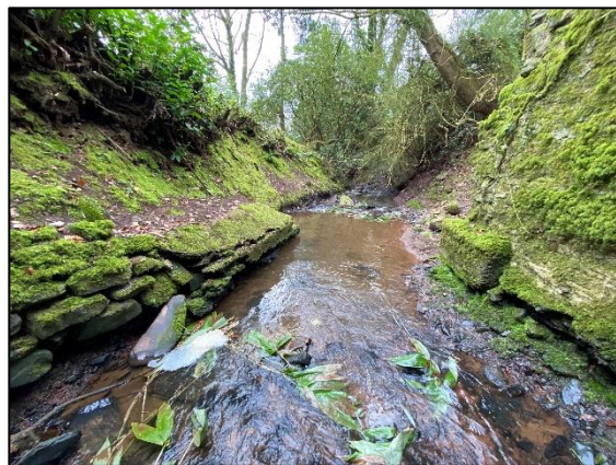
Plate 2: Section of bank (on left) subject to proposed works (facing east)
