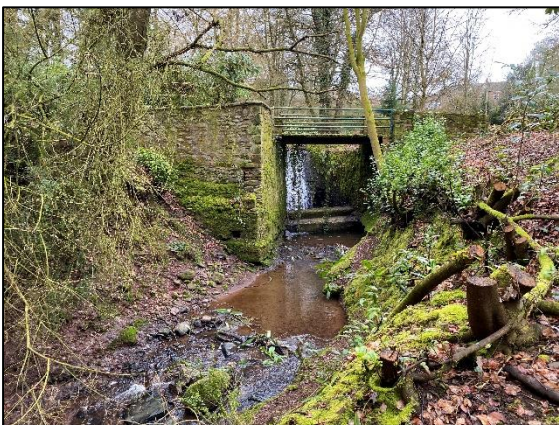
Plate 1: View downstream of the weir (facing west)
