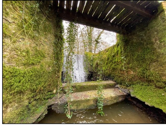
Plate 4: View under the footbridge (facing west)
