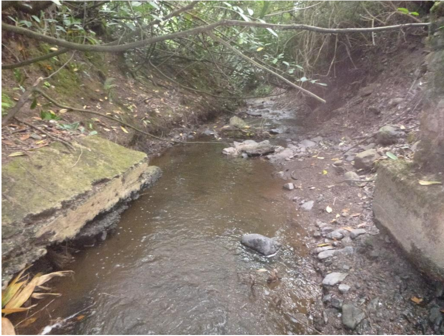
Figure 7: view looking downstream from underneath the footbridge
