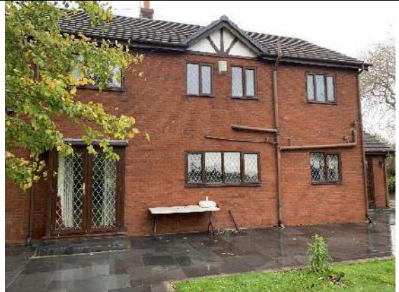
P2: View of the residential dwelling from the south.
