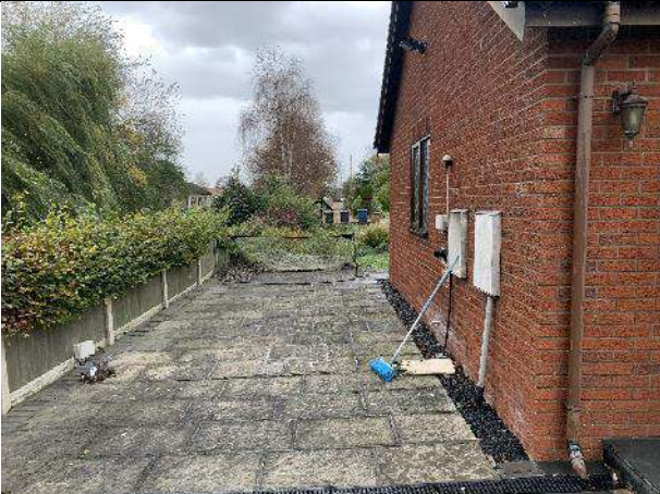
P5: Hard standing flagged ground surrounding the perimeter of the dwelling.
