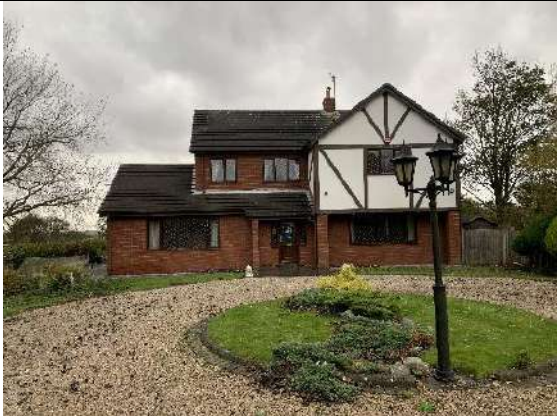
P1: View of the residential dwelling from the north
