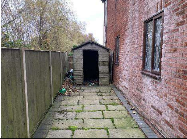
P3: Hard standing flagged area and shed on south-western boundary of the site.
