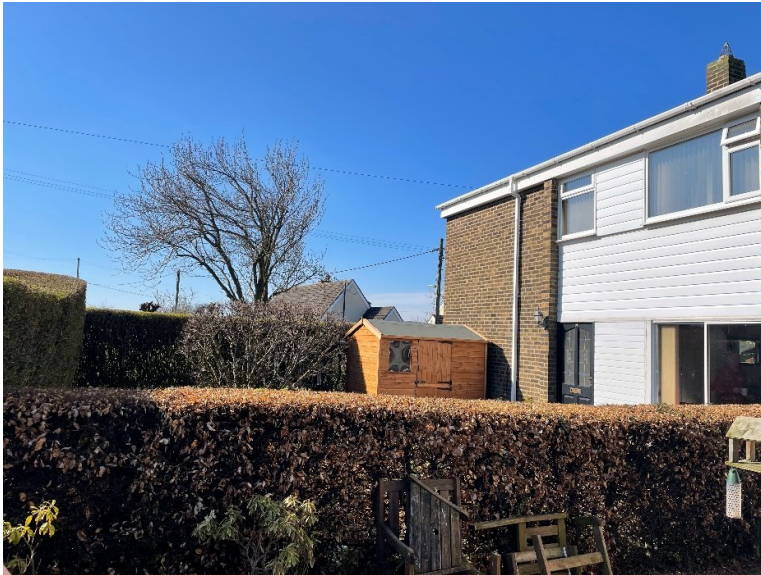
Front of property containing replacement Shed.
