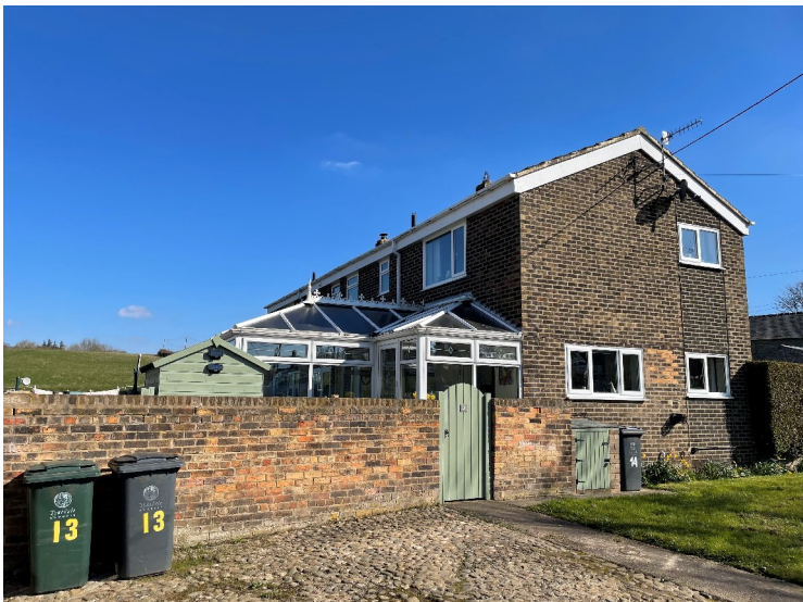
Side of property.
