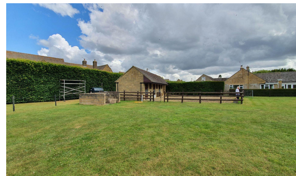
Photograph F: View of existing stables west elevation
