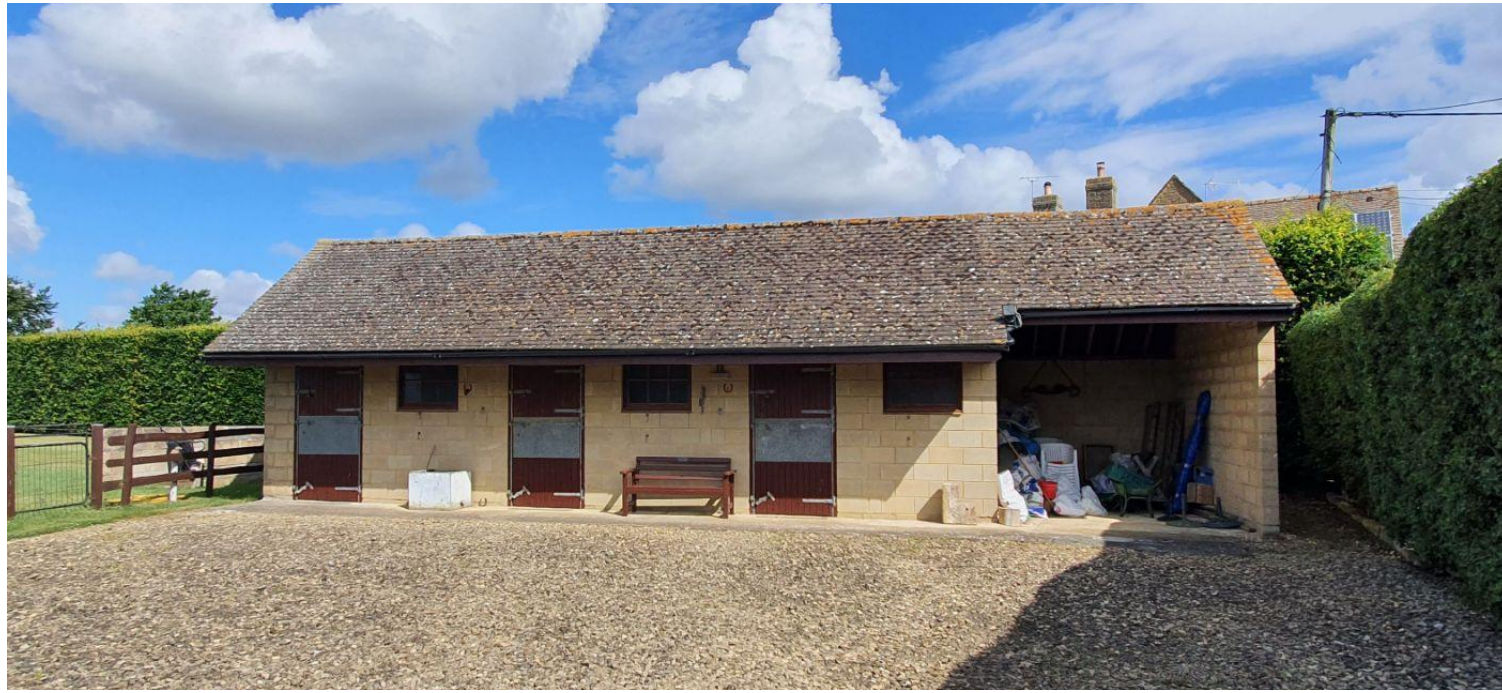
Figure 5: Photograph of southern elevation of existing stables
