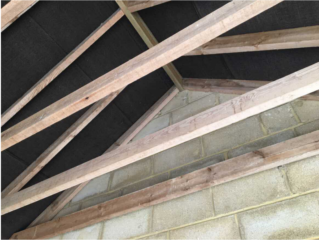
Photograph 5 –Internal view of the roof of the stables
