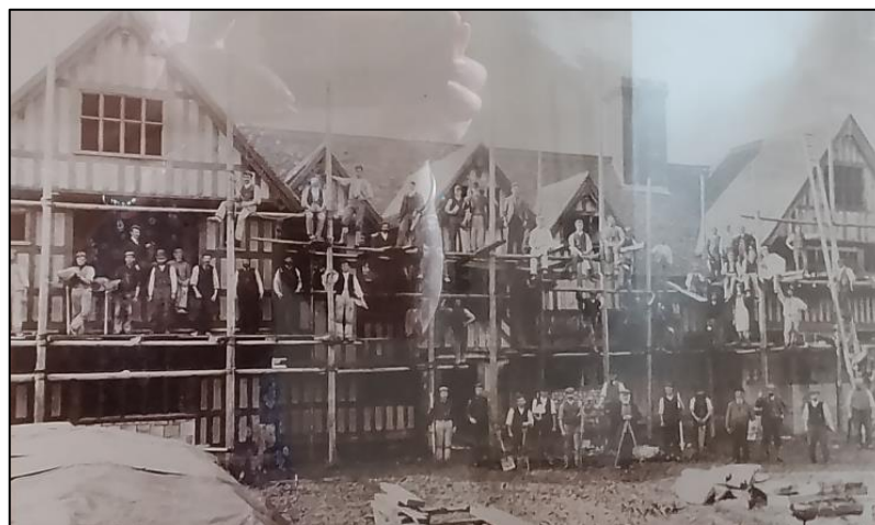
Plate 3. Rumwood Court, repair and extension in progress in the mid-1890s
