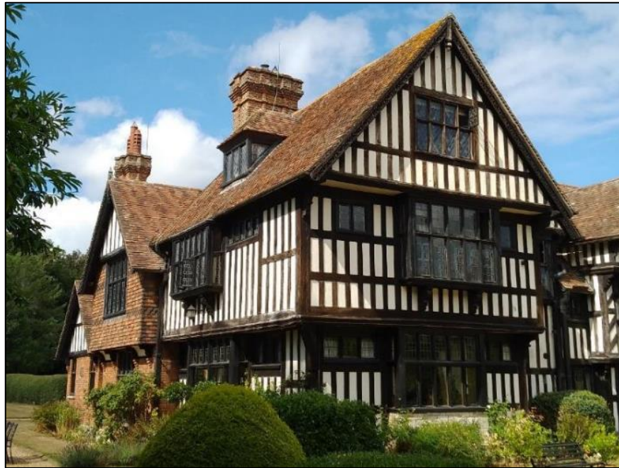
Photo 5. Southeast corner of Rumwood Court; view NW
