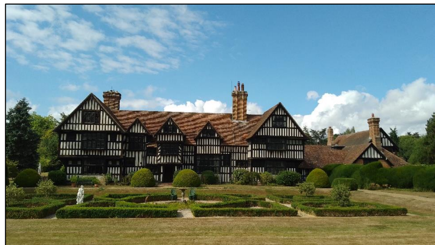
Photo 3. Rumwood Court, east elevation
