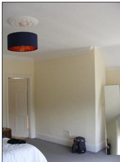
Photo 16. Bedroom 1; south wall chimney breast
