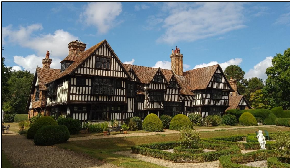
Photo 1. Rumwood Court; south-east corner / east elevation, view west
