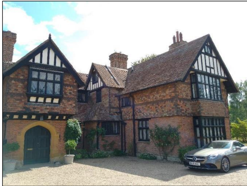
Photo 7. West facing gable of the south wing; view SE
