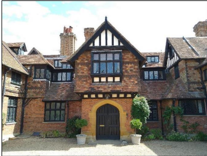
Photo 4. Current main front door; west elevation; view E
