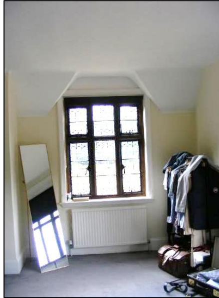
Photo 17. Bedroom 1- South wall window; view south
