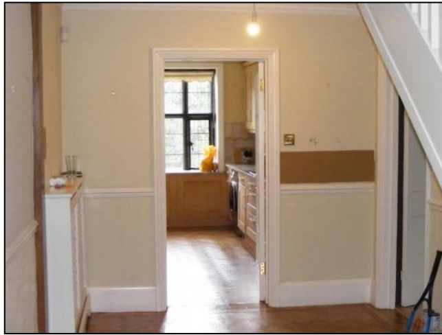
Photo 9. First Floor Hallway; view east towards the Kitchen
