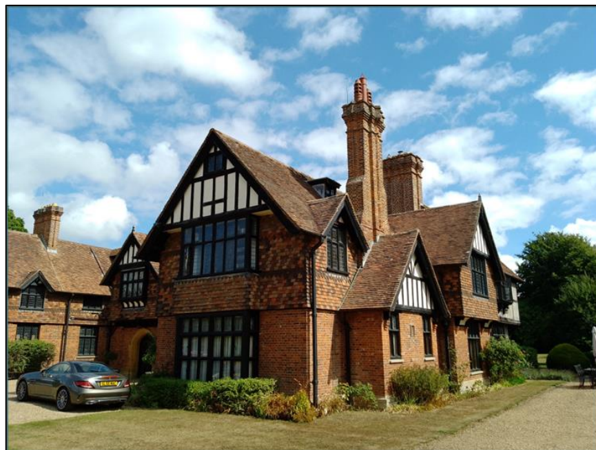
Photo 8. Southwest corner of Rumwood Court; view NE
