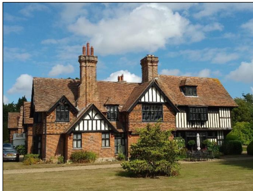
Photo 6. South facing side elevation of Rumwood Court; view N
