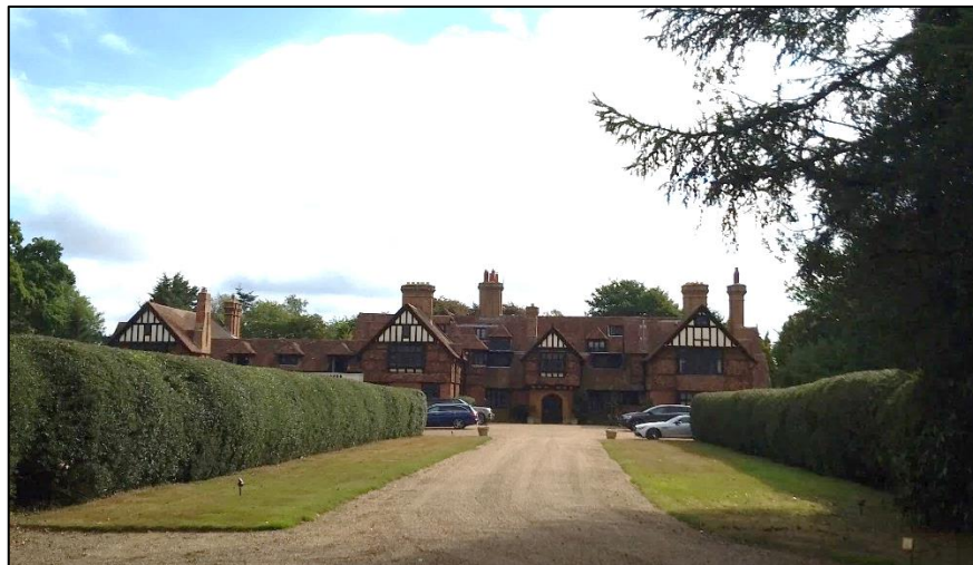
Photo 2. Rumwood Court, west elevation
