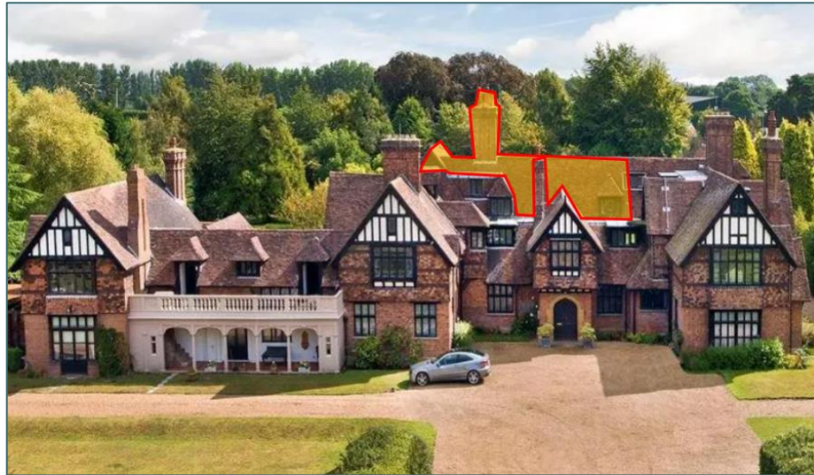
Plate 4. Oblique aerial image of Rumwood Court west elevation
