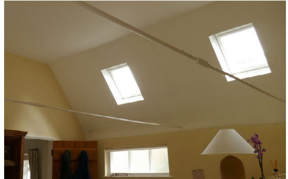
Interior of proposed Kitchen showing steel tie bars and rooflights to be removed. The new Queen Post Truss is to be in the location of wall on the left, and the flat ceiling is the location of collars to be retained.
