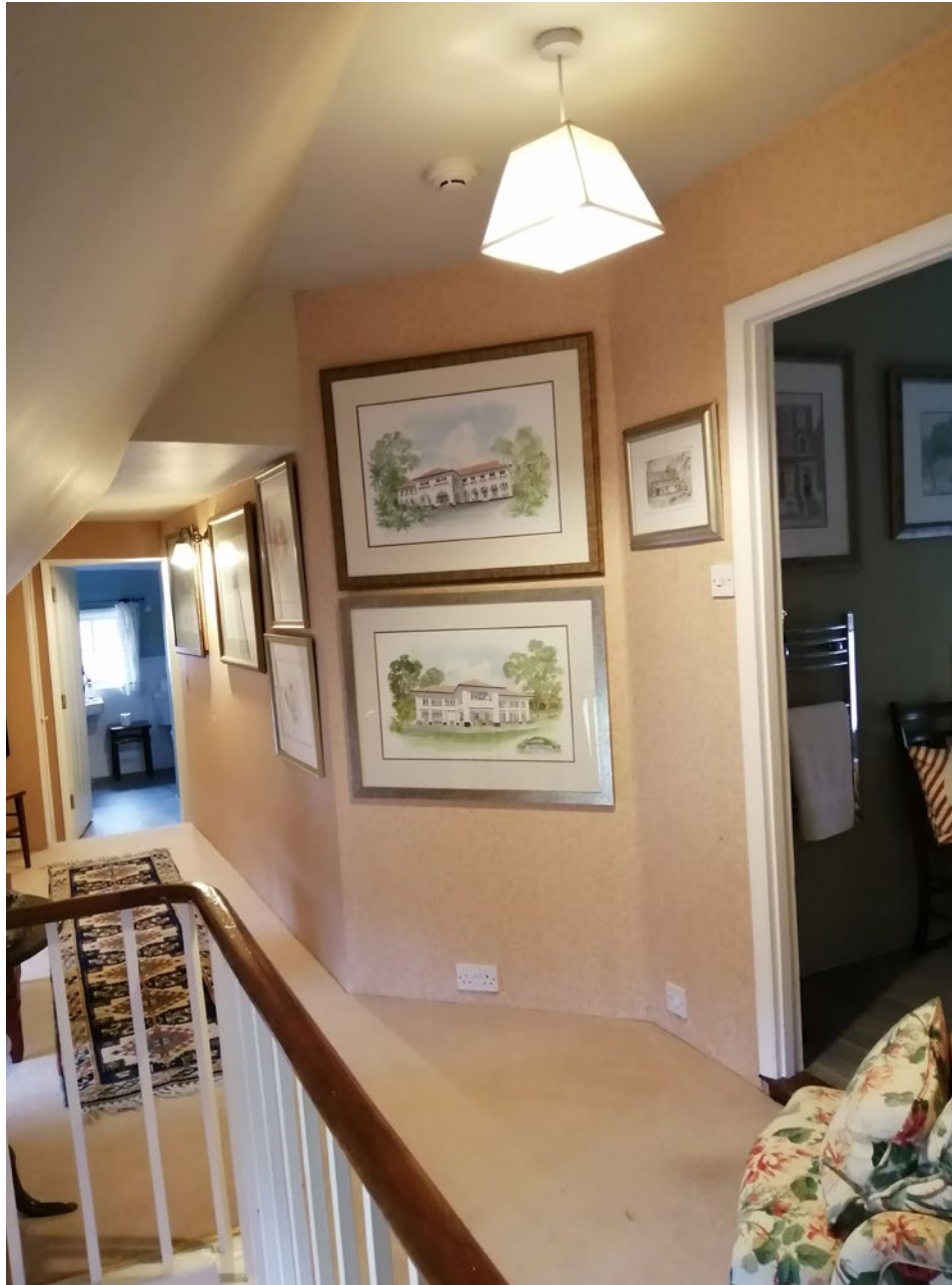
16 & 18 Bedroom Lobby & Upper Corridor- Existing 20th century studwork partition to be replaced in modified location and existing dropped ceiling to be removed
