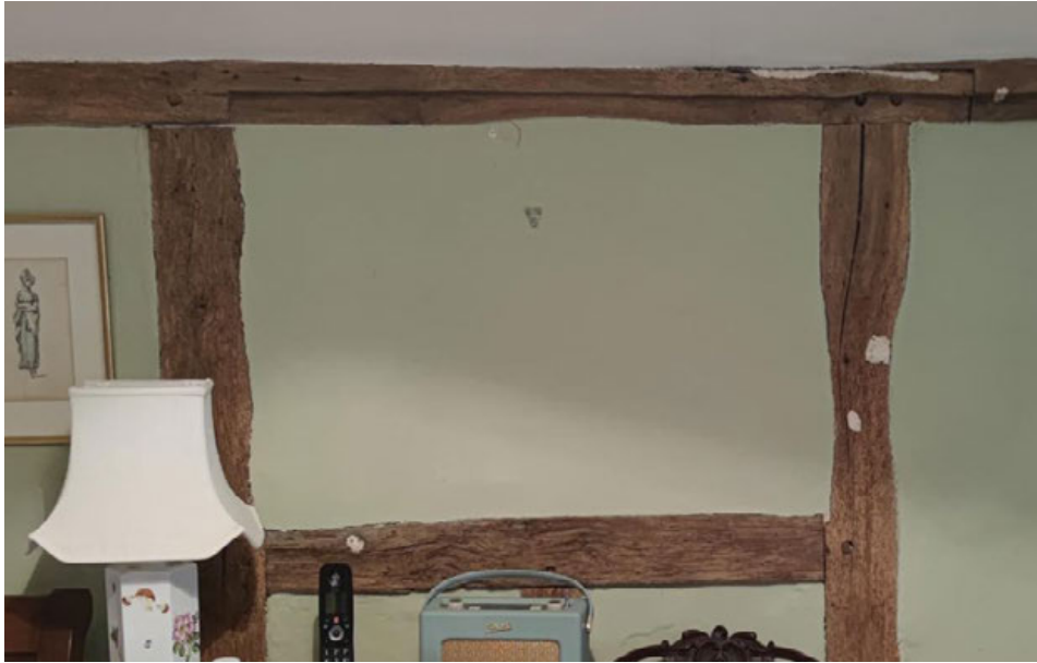
14 Bedroom 1 - Blocked mullion window to be reopened
