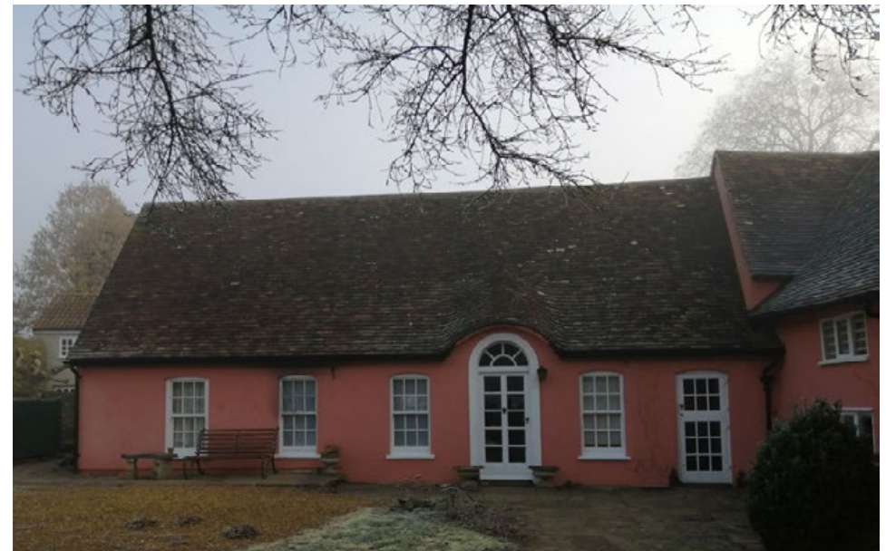
North wing in 2023, viewed from west. Former garage door opening encompasses two left-side windows
