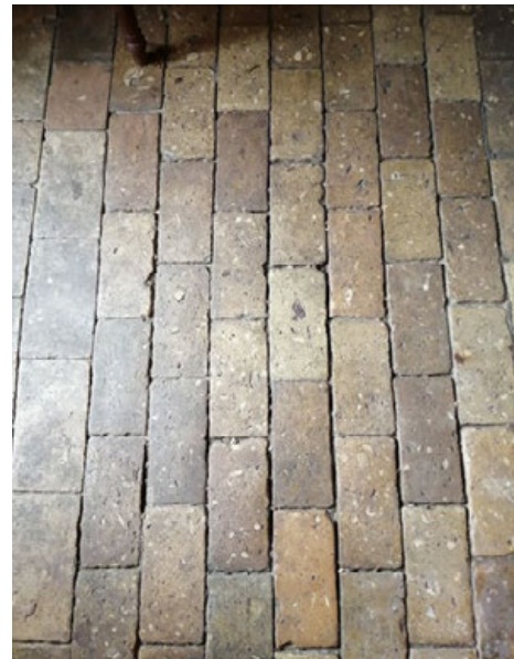
Existing bricks to be set aside and relaid in Back Hall. New bricks proposed for new Back Porch and Utility Room are to be selected to be similar.
