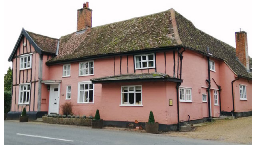
Jackdaws Ford in 2023 showing exposed studwork, concrete ridge tiles over former Butcher's shop and foul drainage pipes on east elevation
