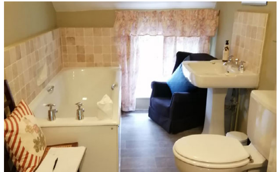
17 Bath 1 - Sanitaryware within Bath 1 to be replaced, including replacement of bath with shower. Existing vinyl floor to be replaced with tiles.
