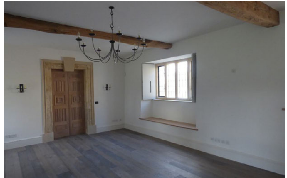
Image showing breathabe woodfibre internal wall insulation and lime render, as approved by Historic England in a Grade I listed building in Lincolnshire
