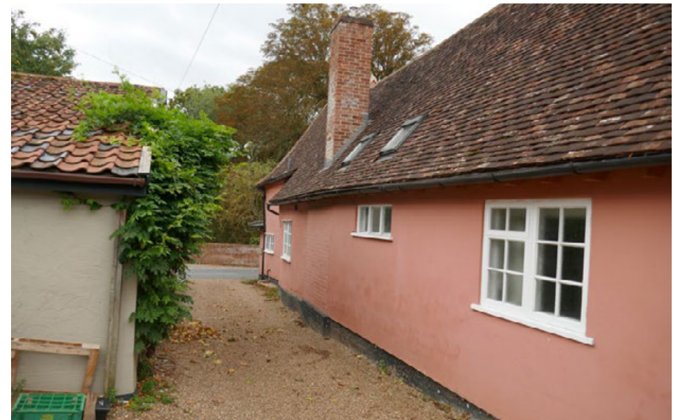
East elevation of Jackdaws Ford looking south towards the street showing rooflights to be removed. The Peacock Inn pub is on the left.
