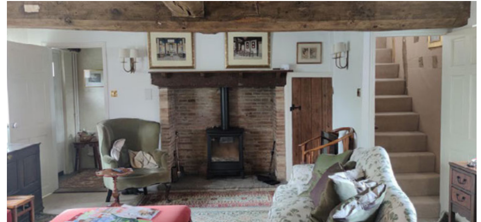
Drawing Room (as seen from the adjacent corridor) showing the existing staircase intruding into the north side of the room
