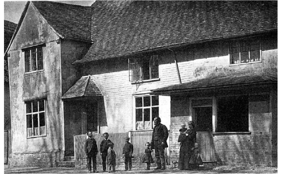
Jackdaws Ford in 1870 showing render finish over exposed studwork, and lead roll hips and gutters over former Butcher's shop (Image published online at Chelsworth.org.uk )
