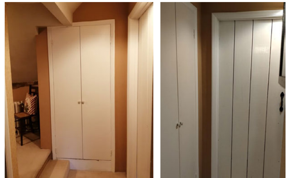
20 FF Lobby - Cupboard to be removed and steps extended. Lobby expanded into previous bathroom space and new stud partitions built as per proposed plan. Existing bathroom door (in image on right) to be moved to new opening in rebuilt partition wall.
