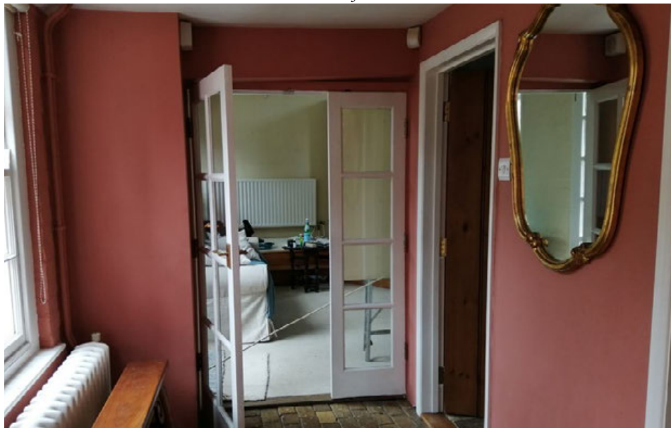
8 Back Hall - Plasterboard partition walls and internal doors to be removed and floor bricks taken up and relaid over new insulated floor buildup
