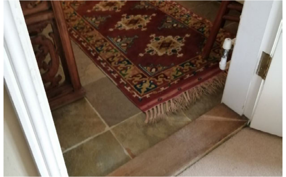
2 Lobby - Modern floor tiles to be removed and replaced with oak floorboards
