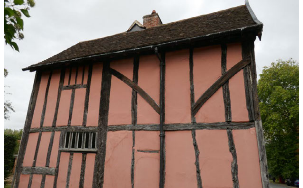
Infilled mullion window on first floor to be reopened
