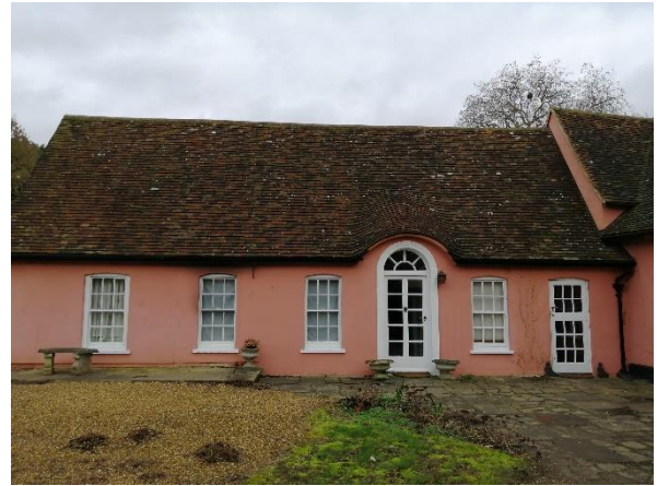
Photo 2: Western façade of northern half of building, showing arched roof over a doorway. To be realigned to match remainder of roof
