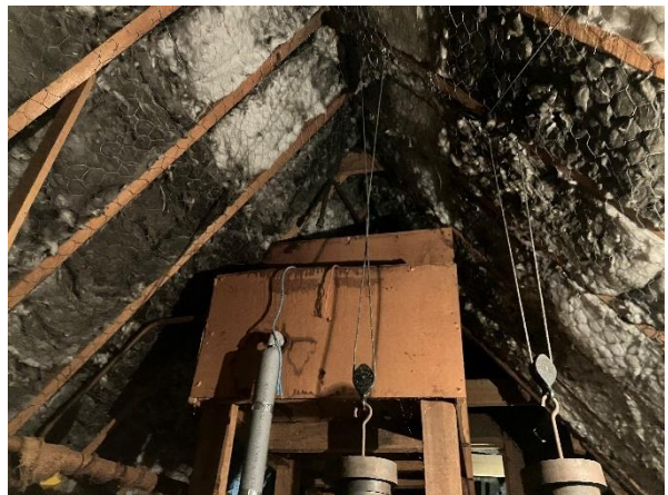
Photo 6: Water tank and insulation between rafters in northern roof space
