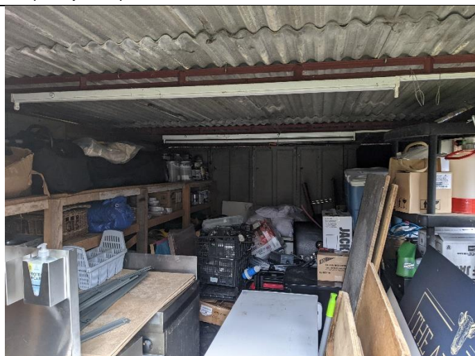
Photo 4 Internal view of the shed
