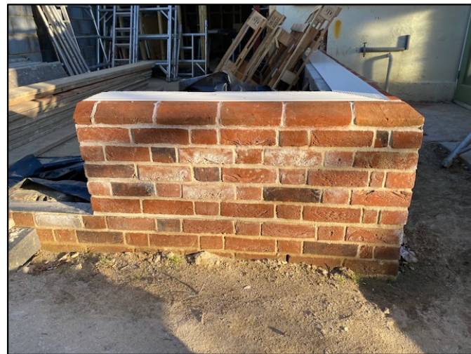
Rear Elevation Plinth Brickwork; Farmhouse Antique Brick from Traditional Brick & Stone
