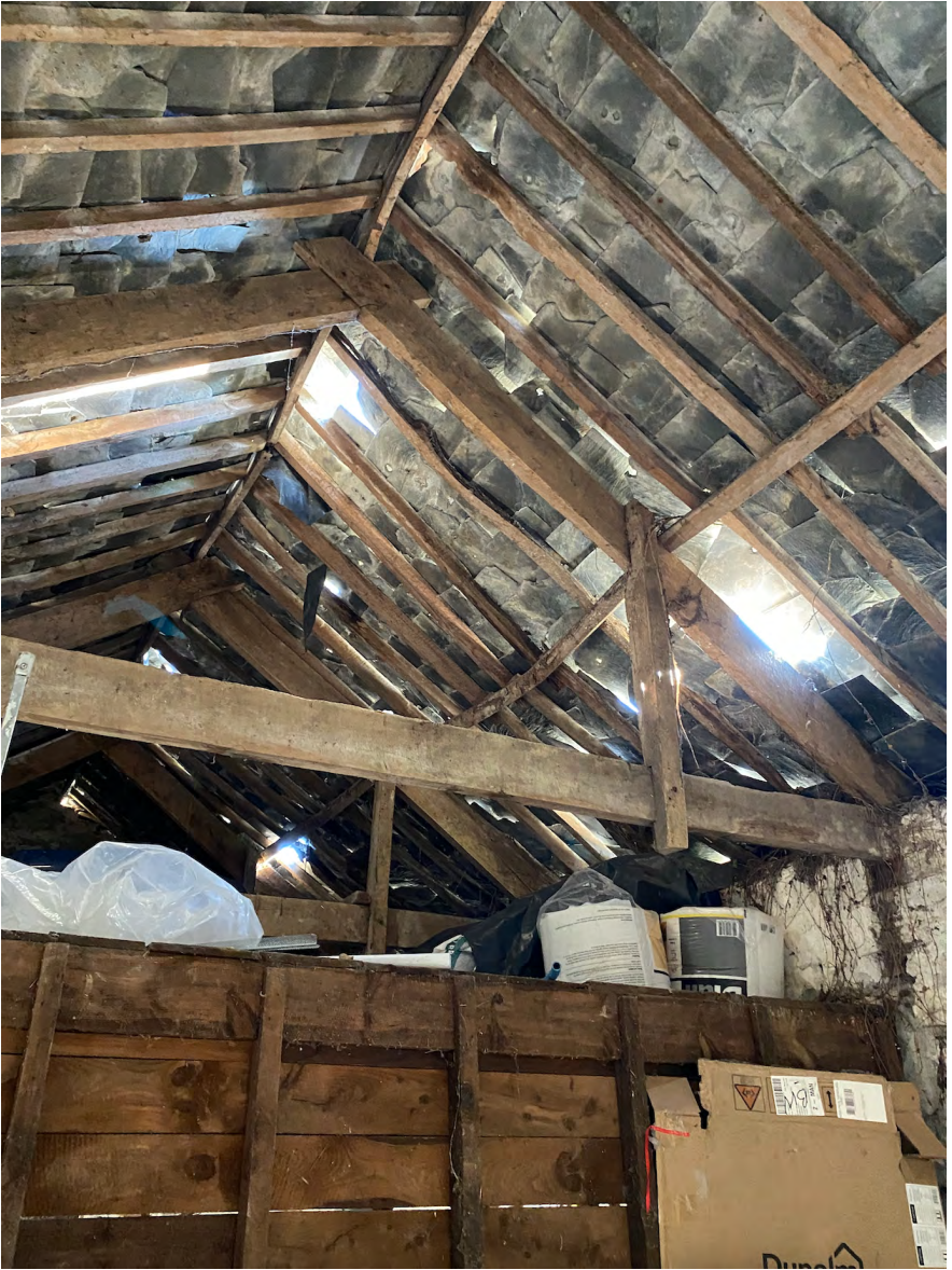
10: BARN INTERNAL ROOF STRUCTURE / PLATFORM
