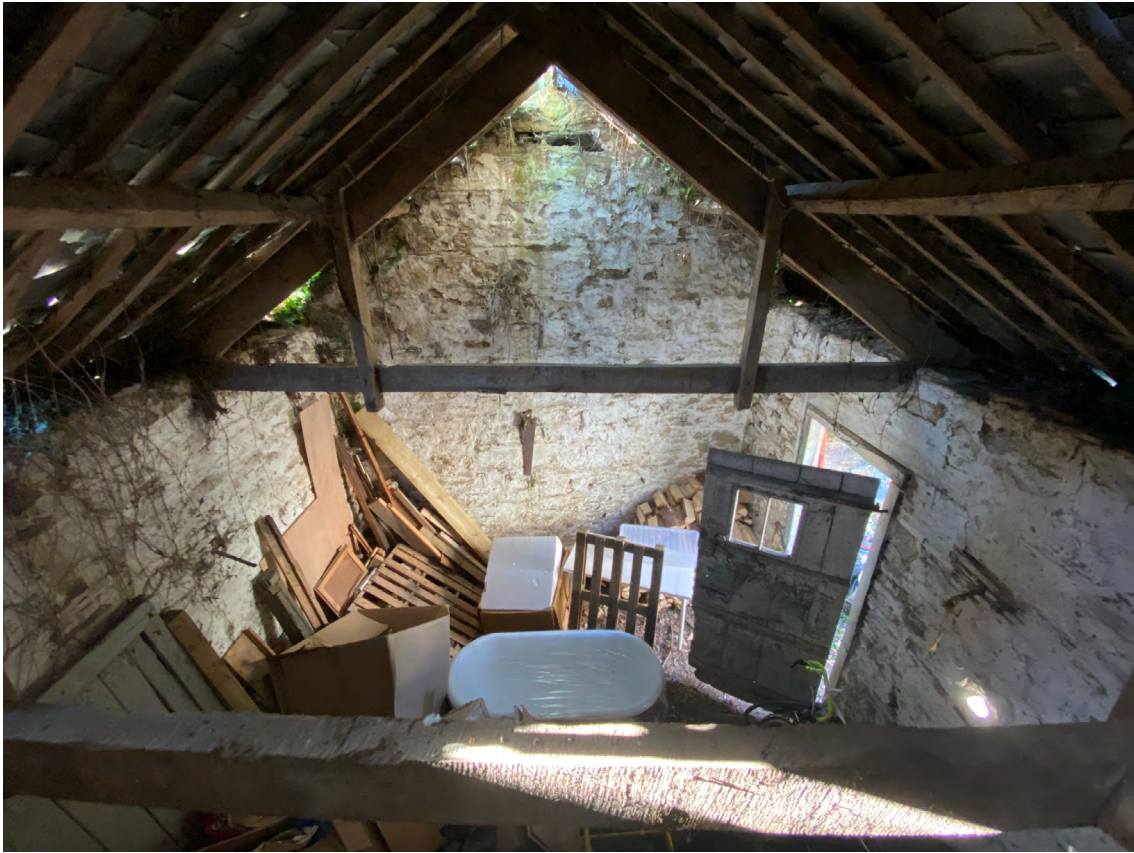
08: BARN INTERNAL FROM PLATFORM
