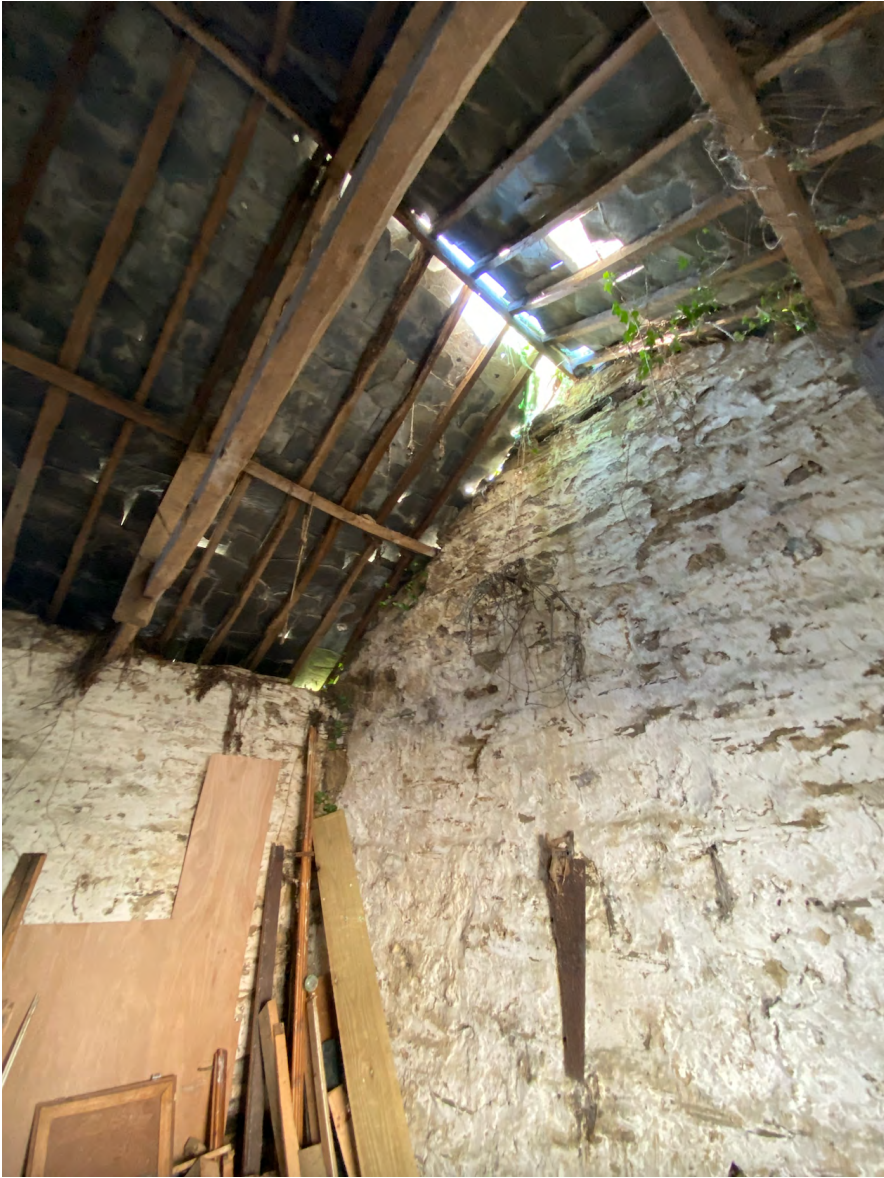
09: BARN INTERNAL ROOF STRUCTURE
