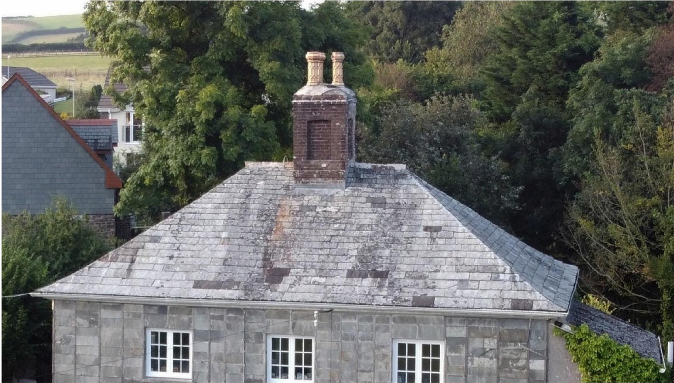
i) Rag slate roof and chimney, souther slope
