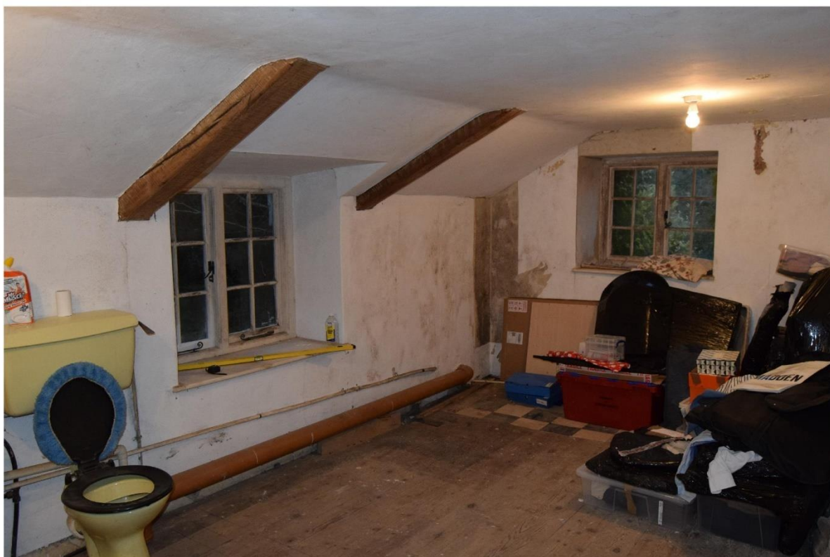
iii) Bathroom looking north east
