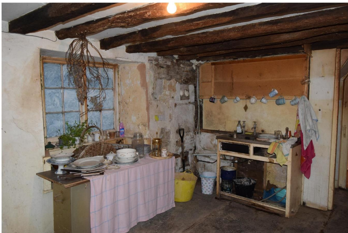
iii) Looking north east towards rudimentary sink unit
