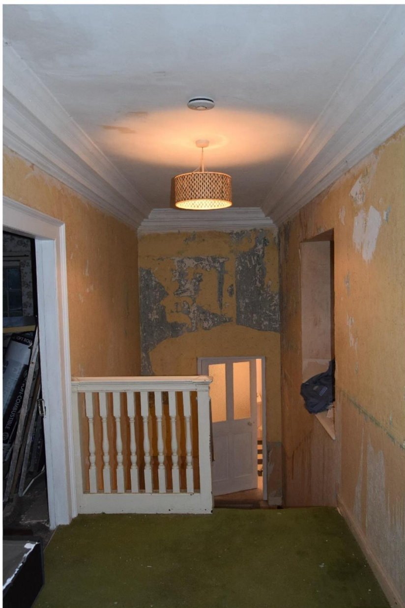
ii) principal stair - looking towards landing - note ornate plaster cornice.
