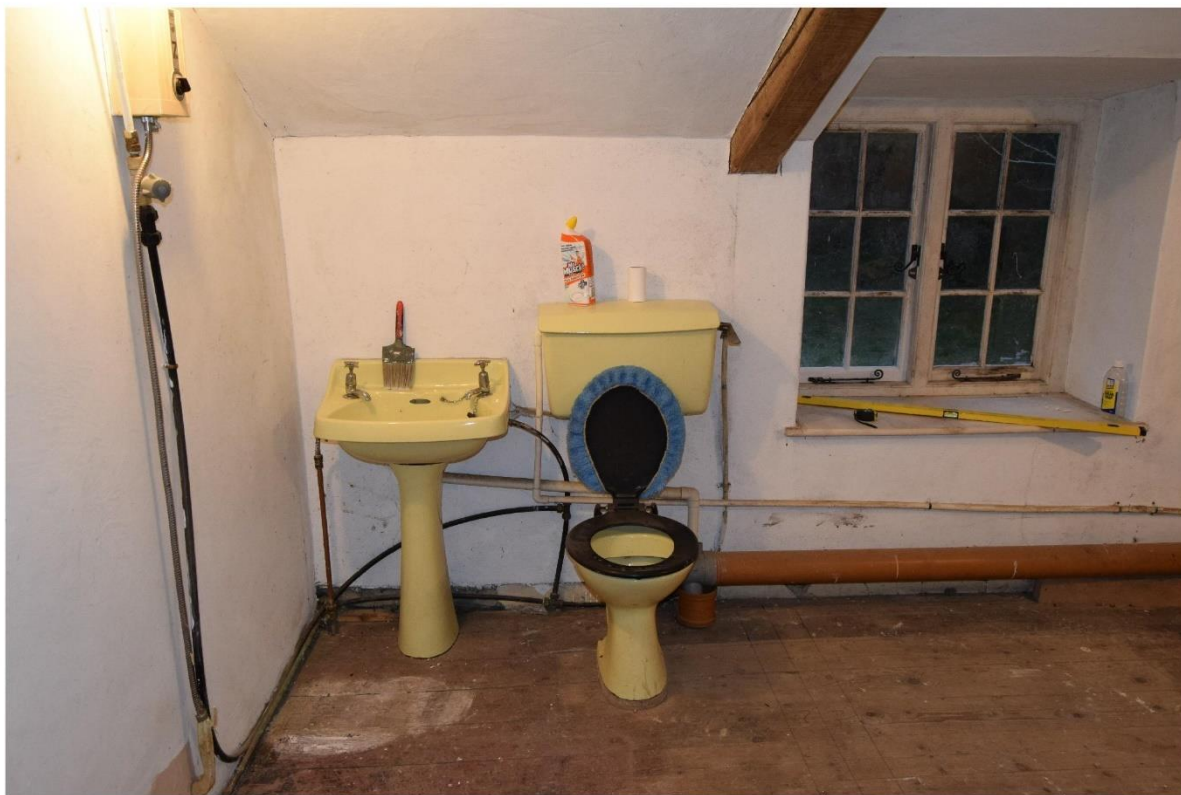
ii) Bathroom - mid 20th century fittings
