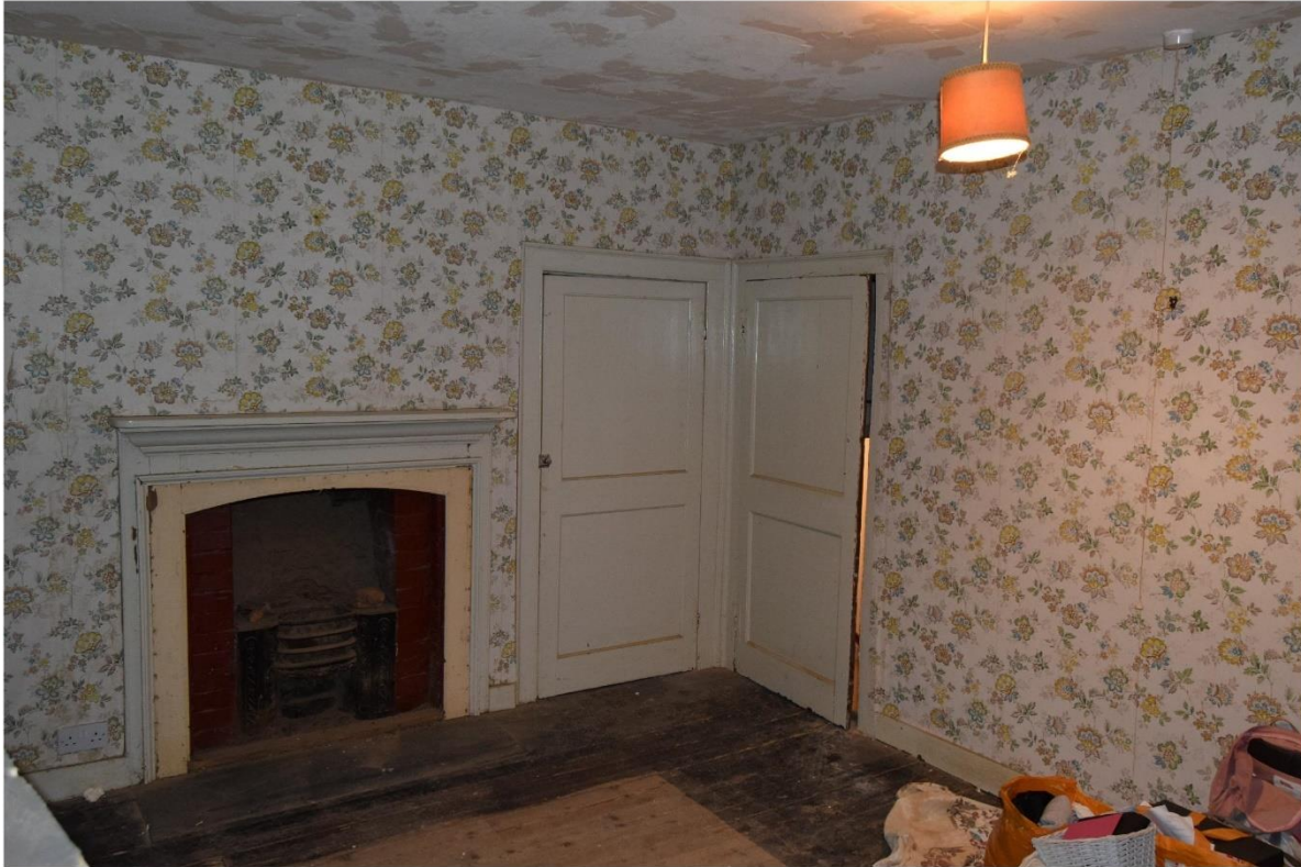
i) Eastern bedroom, looking north west
