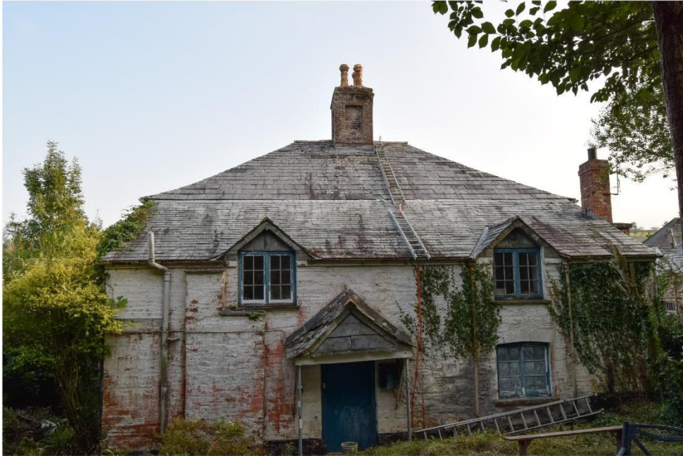
i) North elevation, general
