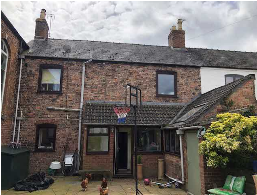
View of the rear elevation of the property
