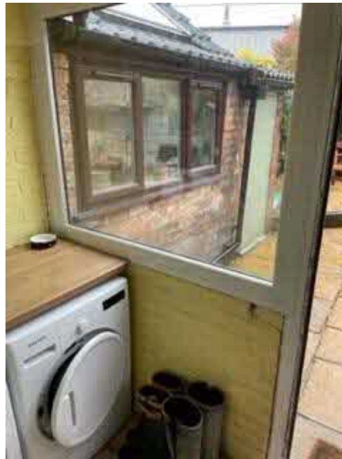
View of the single brick thick wall construction forming part of the extension
