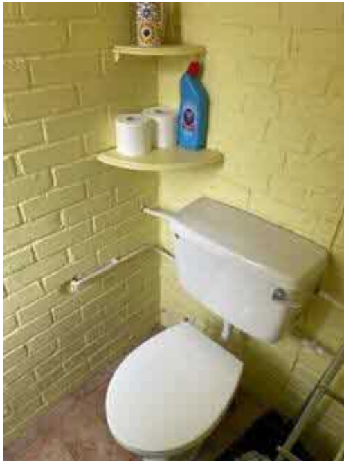
View of the single brick thick wall construction forming part of the extension
