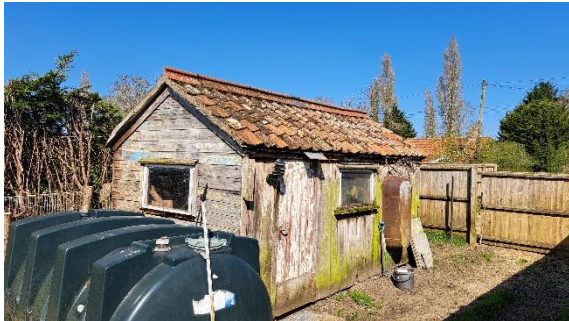
Photo 7 View from south east of Shed
