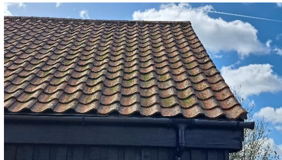
Photo 2 View of roof section showing location of proposed flue
