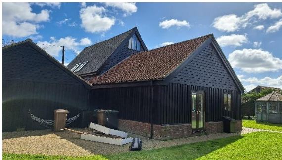
Photo 1 View from NW of NW corner of barn extension showing area of proposed works
