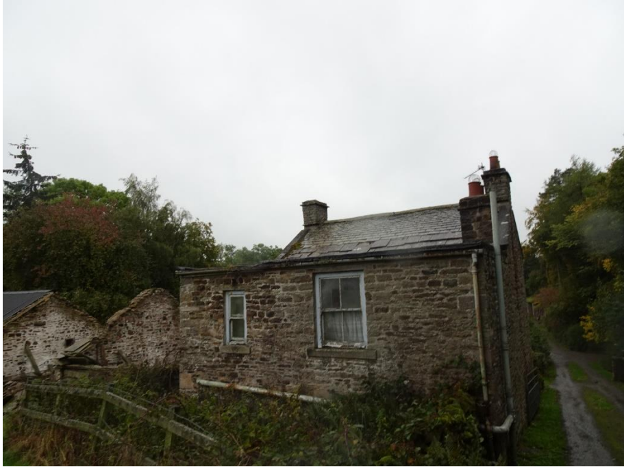
Photo 2 – Cottage North elevation
