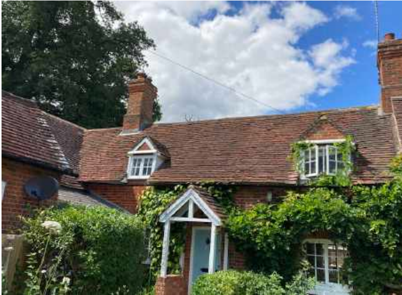
The Main Façade
