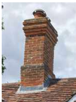
Chimney 1: Front View
