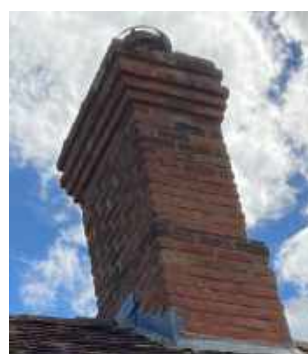
Chimney 1: Rear View
