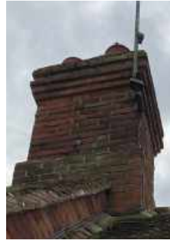
Chimney 2: Rear View
