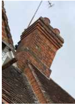
Chimney 2: Front View
