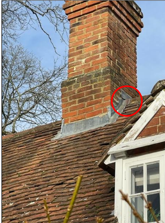
Photograph 13: Lifting around lead flashing.
