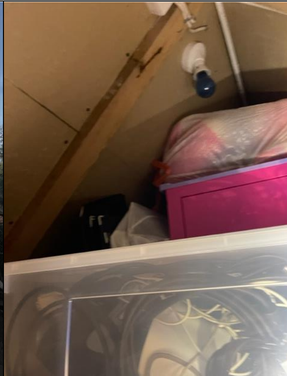
Photograph 10: Loft space used for storage.
