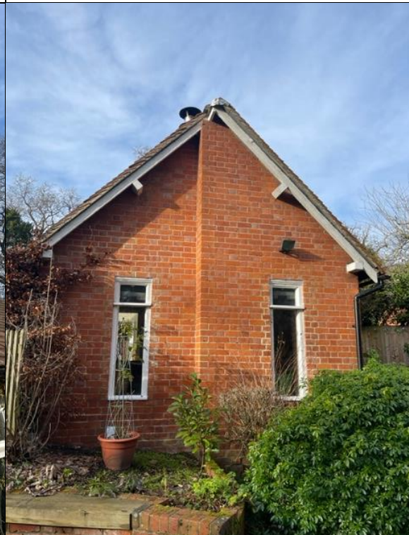
Photograph 8: Side elevation with wooden barge boards
