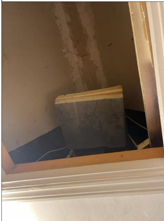
Photograph 11: Loft space used for storage.
