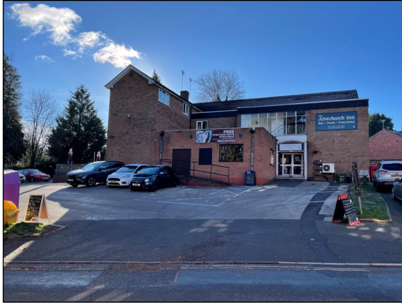
Figure 15: View of the front of Alvechurch Sports and Social Club.
