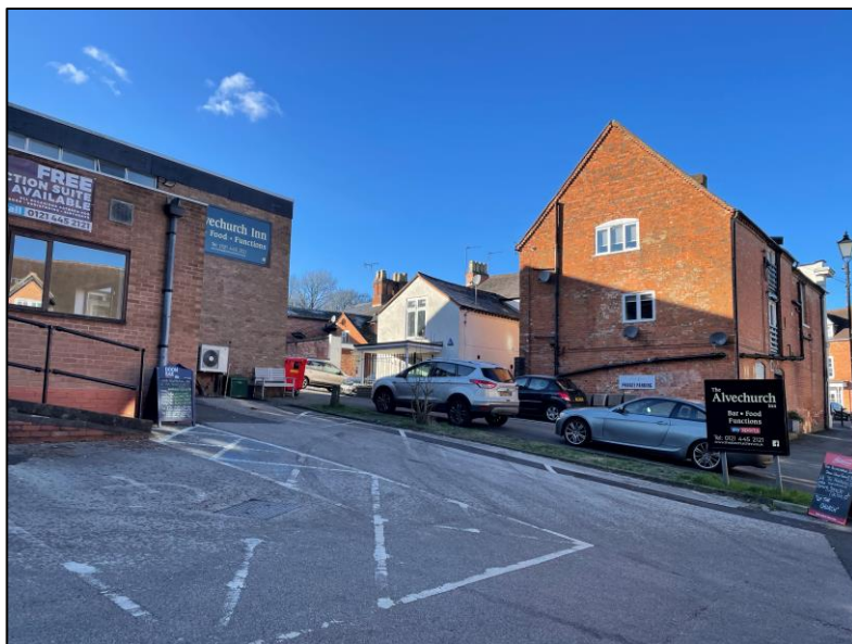
Figure 17: View to the rear of properties facing The Square.
