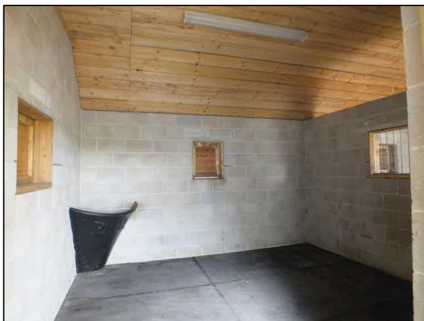
Fig 7: A typical view of the interior of the stables.
