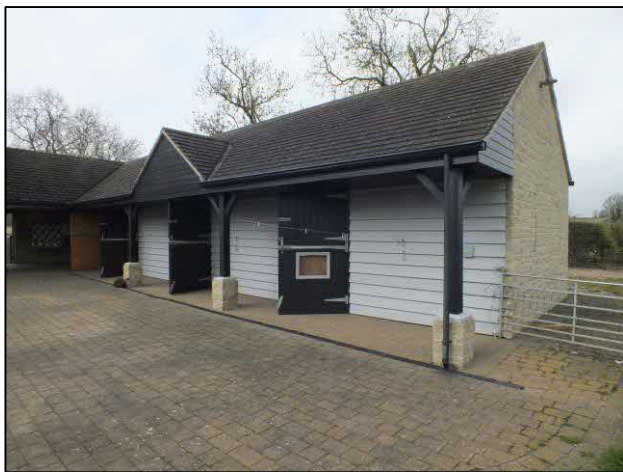
Fig 5: The exterior southeast face of the stables
