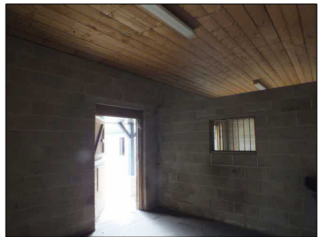
Fig 8: A typical view of the interior of the stables.
