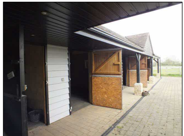
Fig 6: The southeast face from the tack room area.
