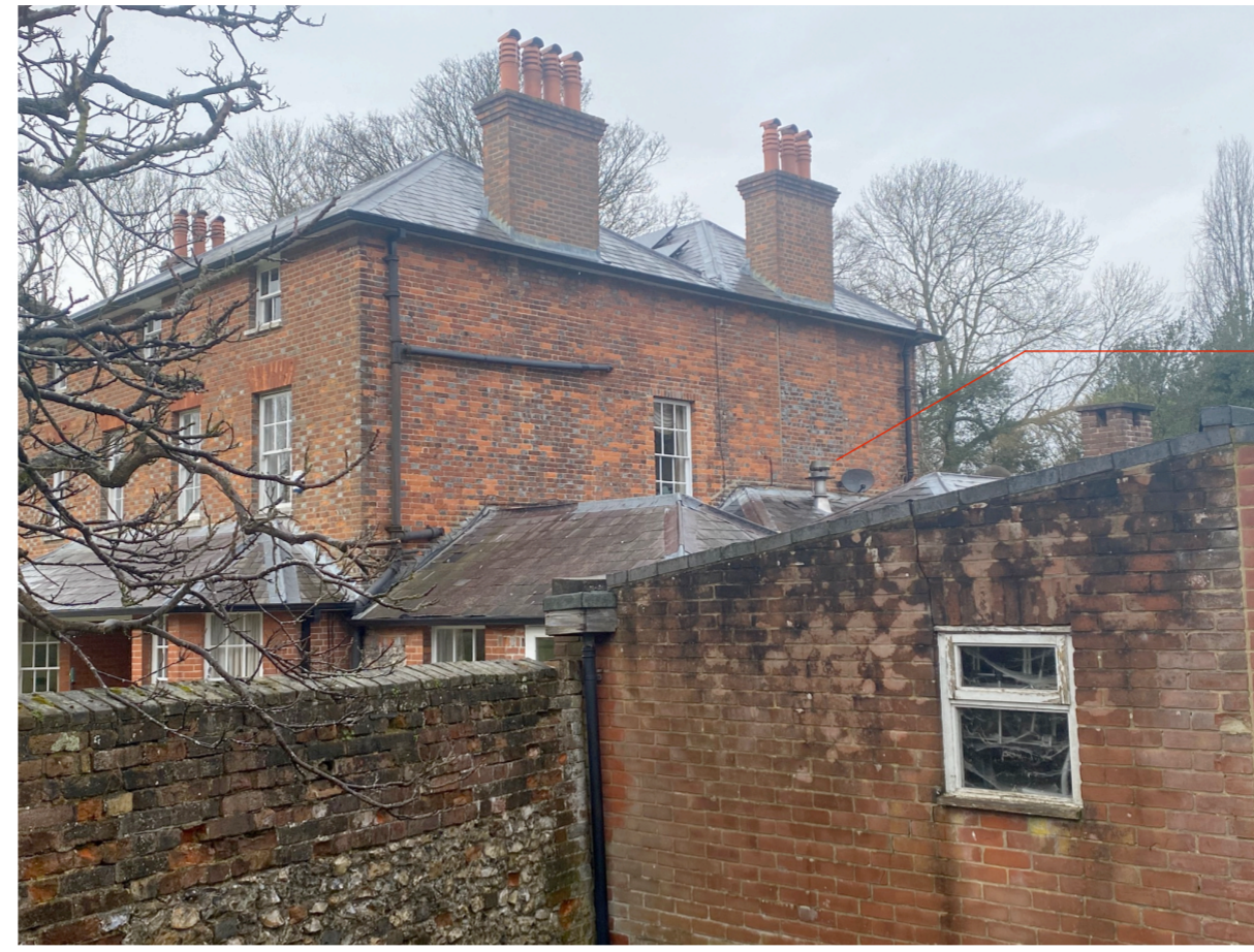
IMAGE OF ELEVATION OF EASTERN GABLE WALL
